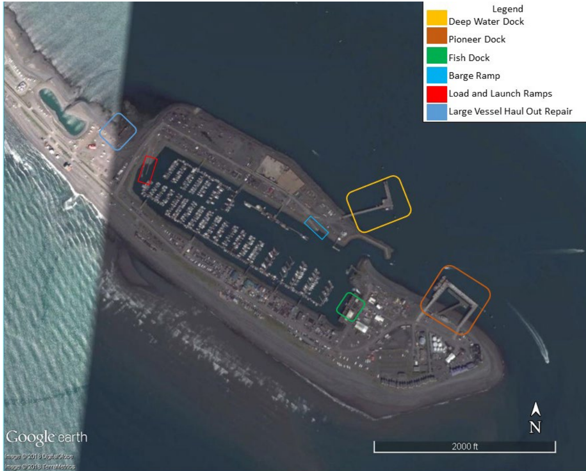
Figure 5. Port of Homer Facilities
