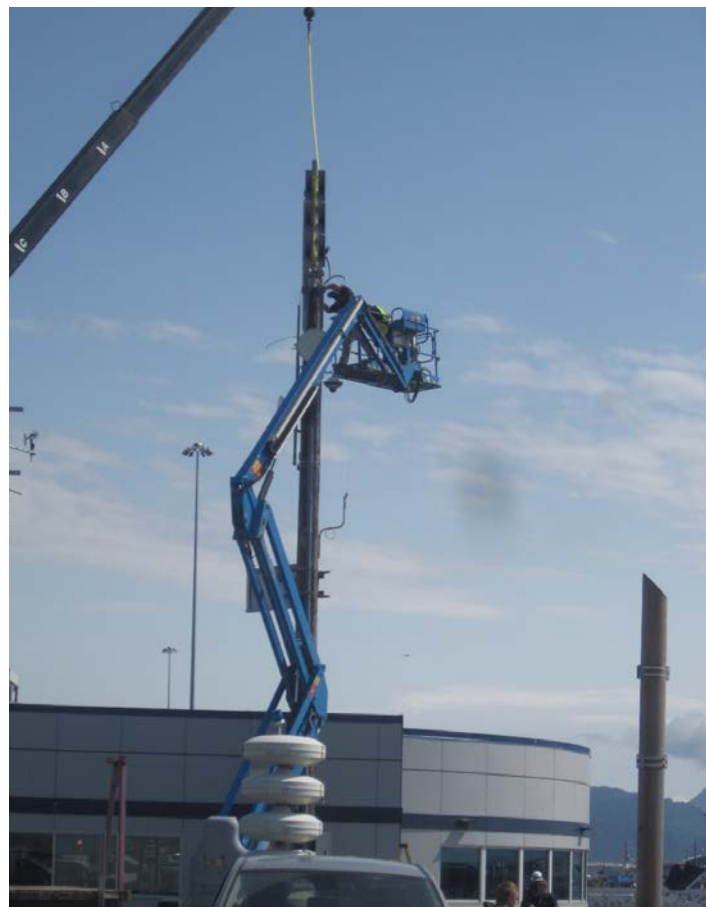
The KPB's tsunami tower rebuild team installed the new tsunami warning system on the pole next to the Harbormaster's office.
