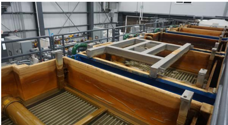
Membrane Filters at Water Treatment Facility
