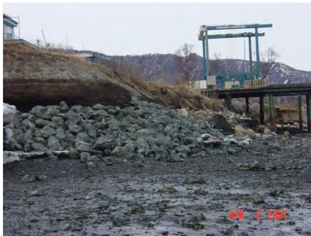
Photo 4: Homer bluff private property riprap project April 2007
