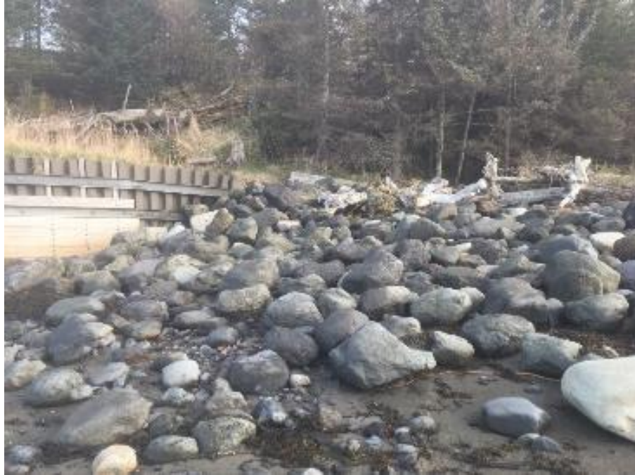
Figure 5. Observed armor stone at east terminal of the seawall.
