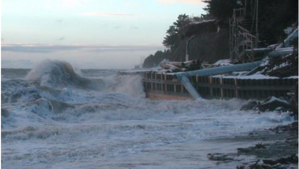
Figure 7. Storm waves impacting existing Homer seawall (photo courtesy of City of Homer).
