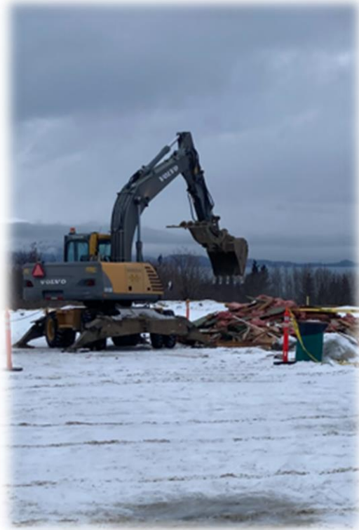
1. KHP Restroom Demolition
