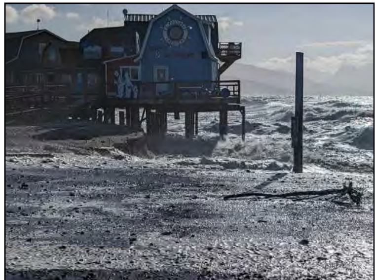
Example of recent active erosion on the Homer Spit. City Manager at 235-8121
