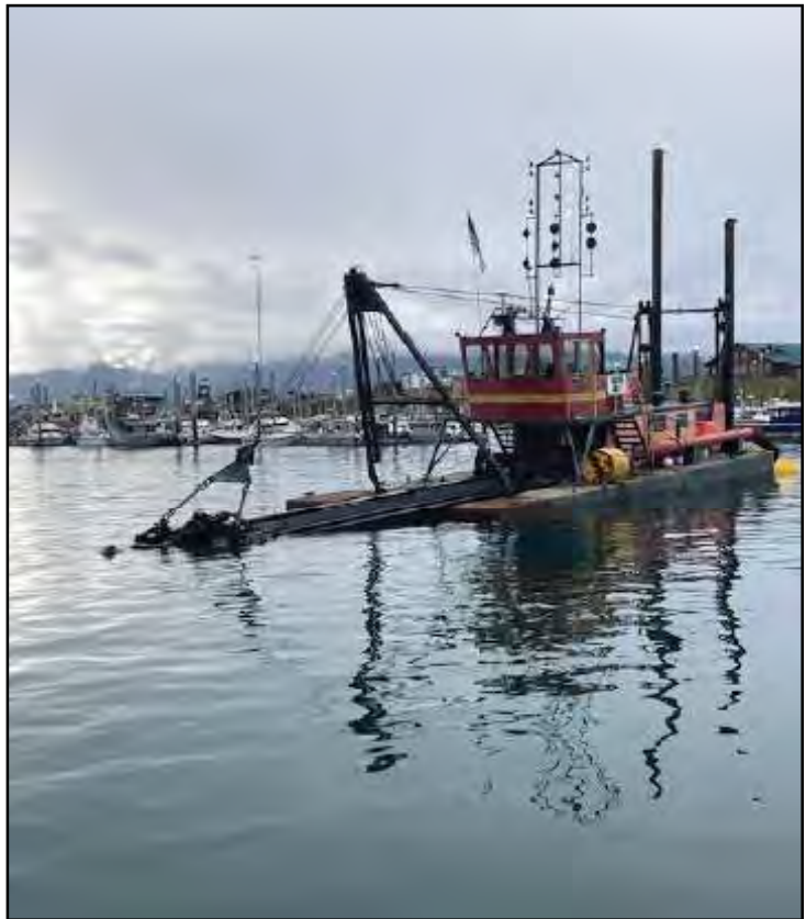
A dredge in Homer Harbor during the US Corps of Engineer’s annual dredging of the harbor’s navigable channel.
