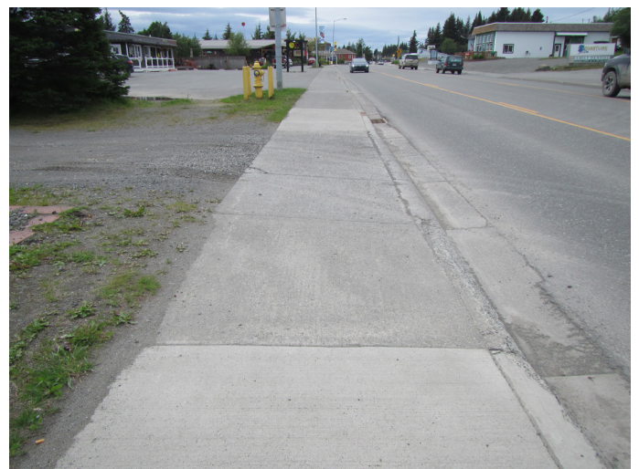
Figure 20: Driveway Entrance with Steep Cross Slope
