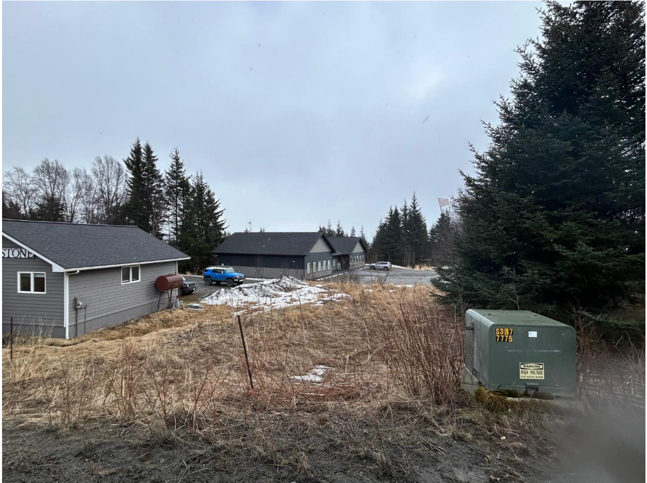
Existing Buildings #1 and #2 on the 2.33-acre parcel
