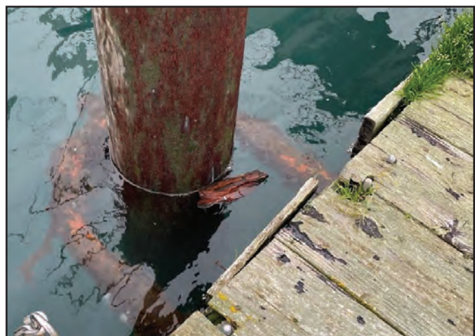
Low freeboard resulting in submerged pile collar.
