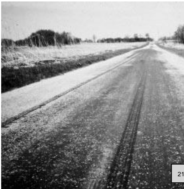
▼ Severe flushing.
