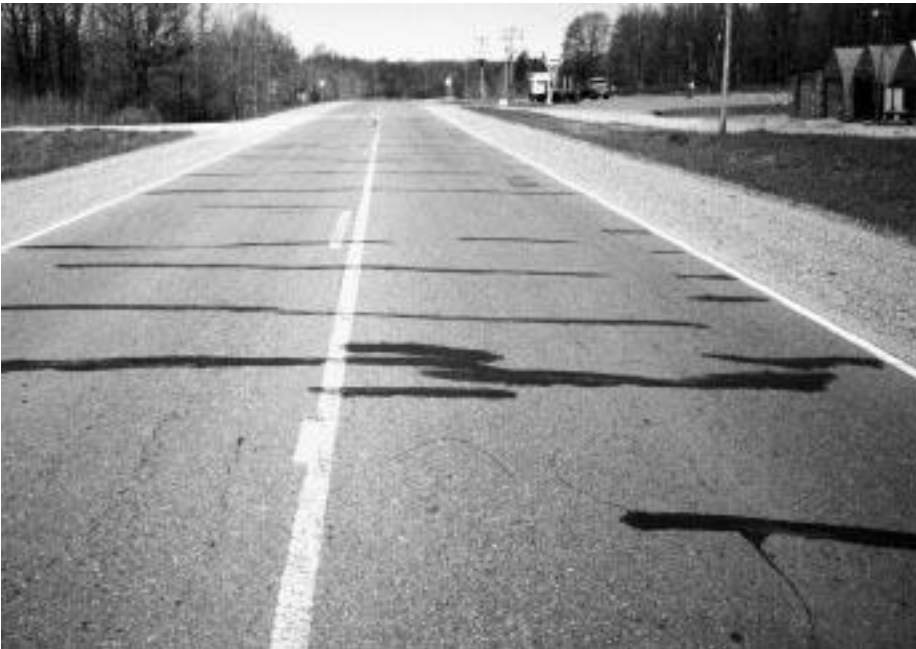
◀ Sealed cracks, a few feet apart.
