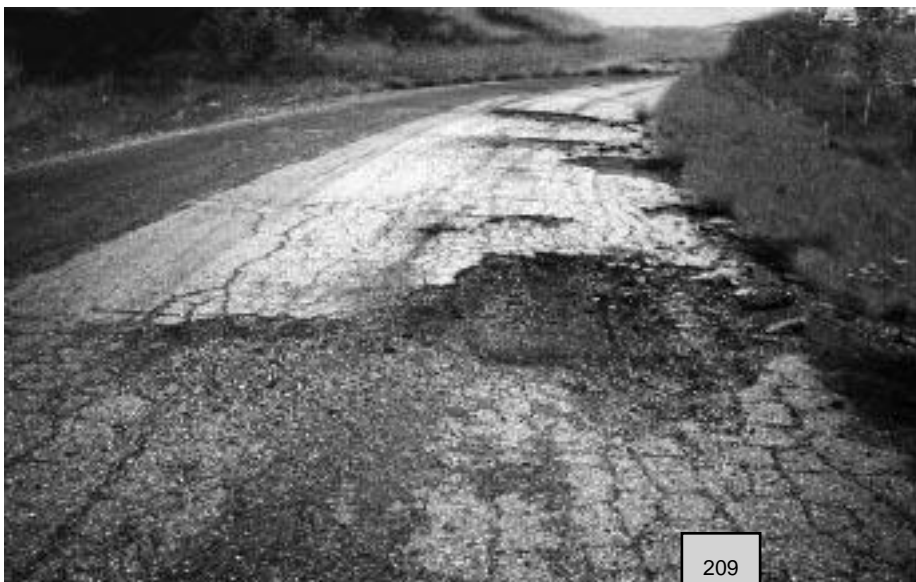
◀ Large, isolated pothole, extends through base.
