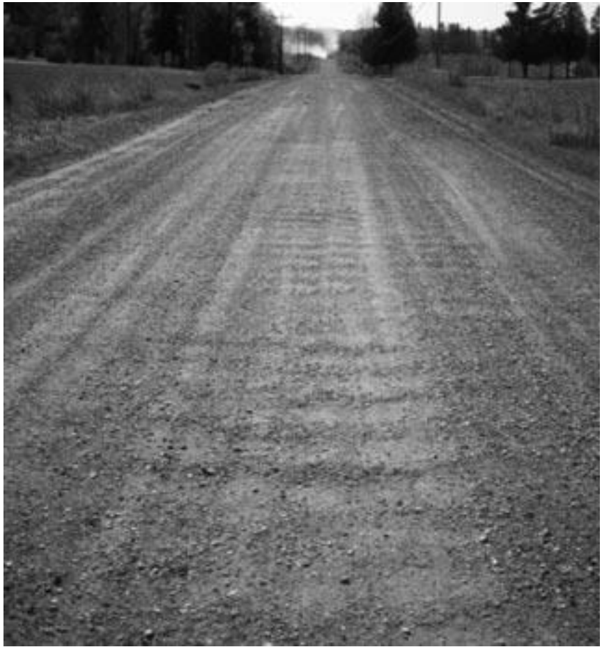
▼ Moderate washboarding in center of road.
