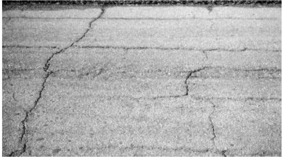
▼ Block cracking with open cracks.
