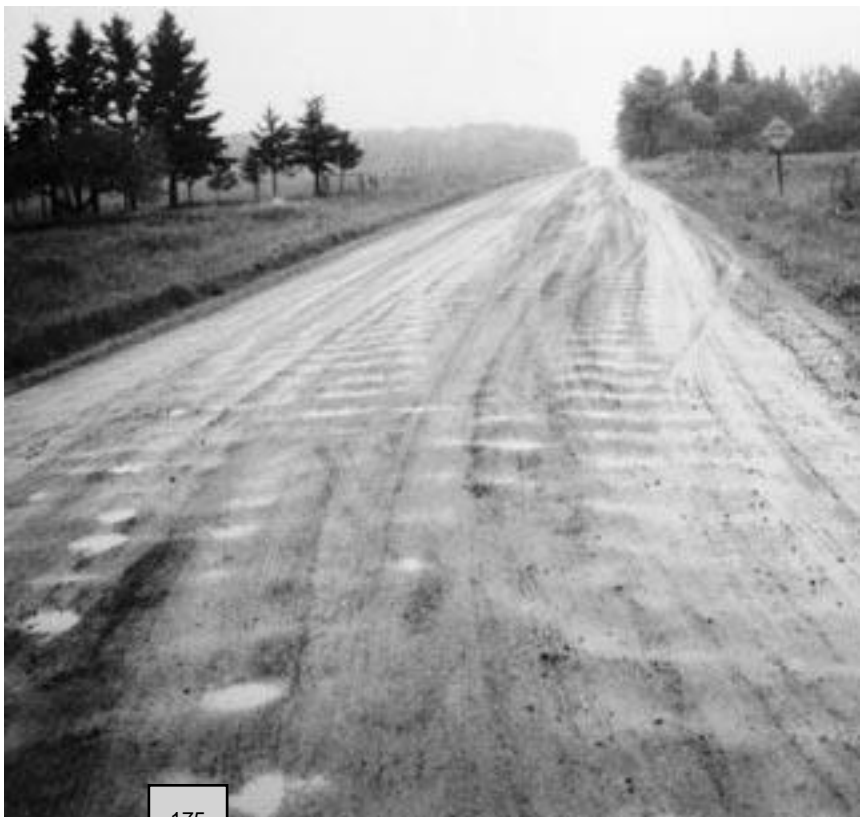
► Severe washboarding traps water.
