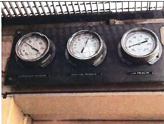
5. Intermediate Pressure (35 psi), Discharge Pressure ( 165 psi) and Low Pressure Gauges (0 psi)
