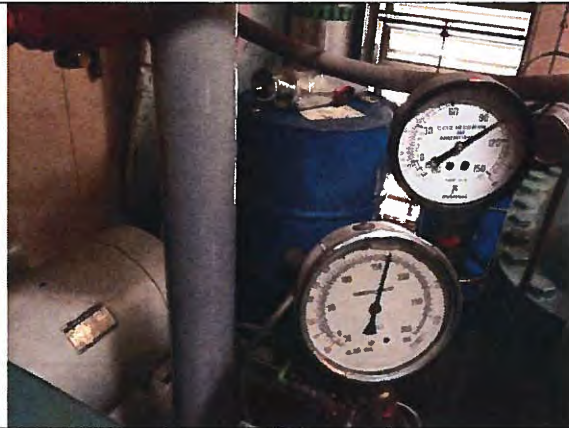
4. #4 Typical High Stage Compressors Pressure Gage (103 psi) and (90 psi)
