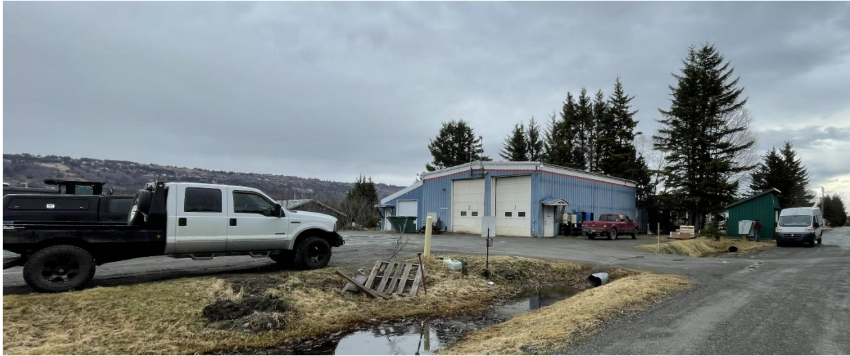
View of existing building from Bay Ave looking north.
