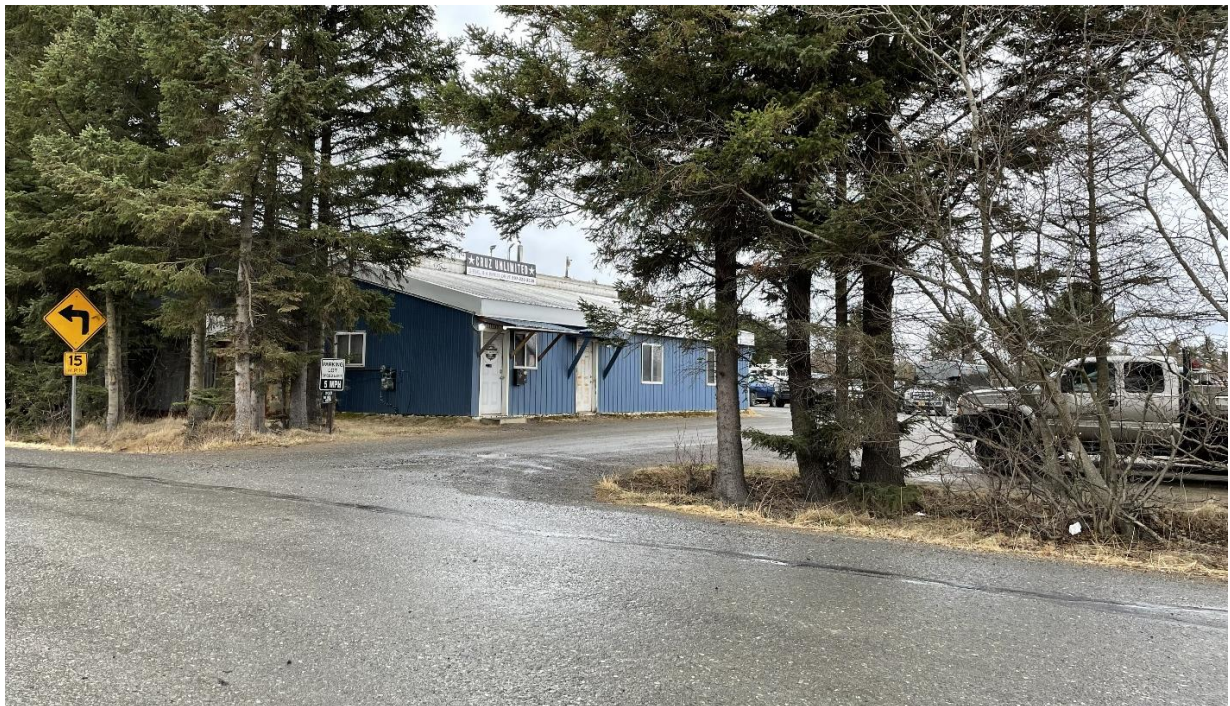
Existing building located at 3267 E Street.
