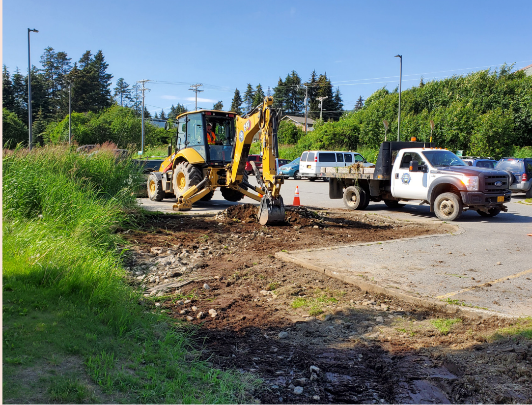
Staff from Public Works dredged out the drainage channel on the south side of the parking lot on August 15
