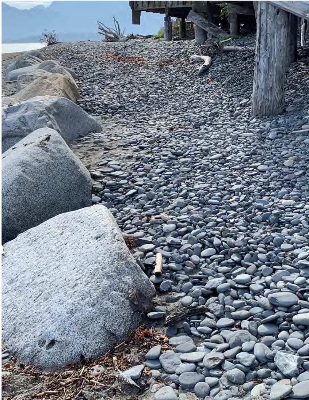
Figure 8. Boulders placed along Land's End.
