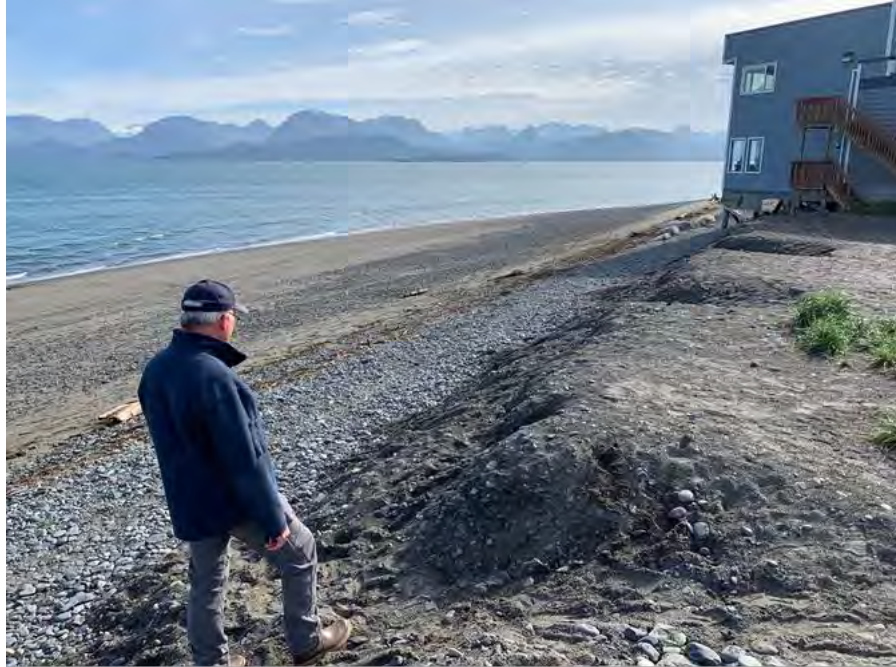
Figure 6. Escarpment along Spit demonstrating natural sorting of placed dredged material.
