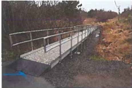
ADA ramp on Poopdeck Extension Trail
