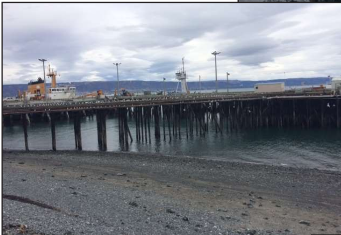
The former Main Dock in Homer's Port & Harbor is over fifty years old, defunct and deteriorated to the point that it is a hazard and a liability.
