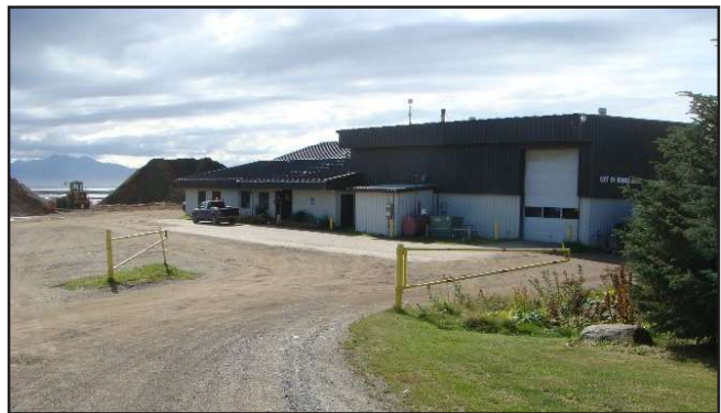
City of Homer existing Public Works facility.
