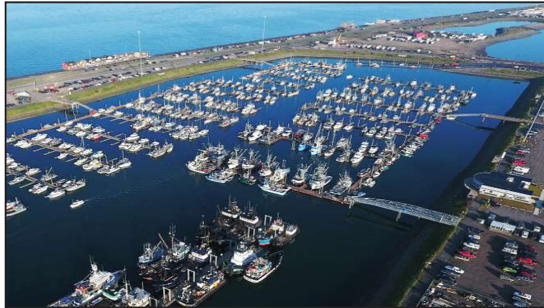
System 4 floats to be replaced.
