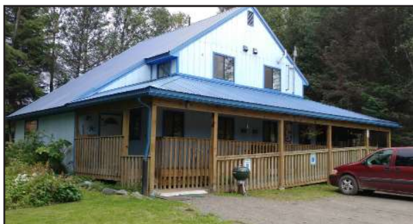
Annual maintenance to the Annex, an older, former residential building that houses several SPBHS programs, often exceeds SPBHS' entire agency maintenance budget.
