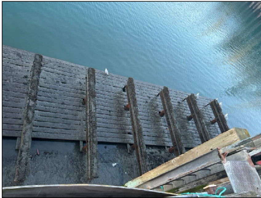
Figure 1-4. Photograph of Primary Beams and Decking Taken from Pier
