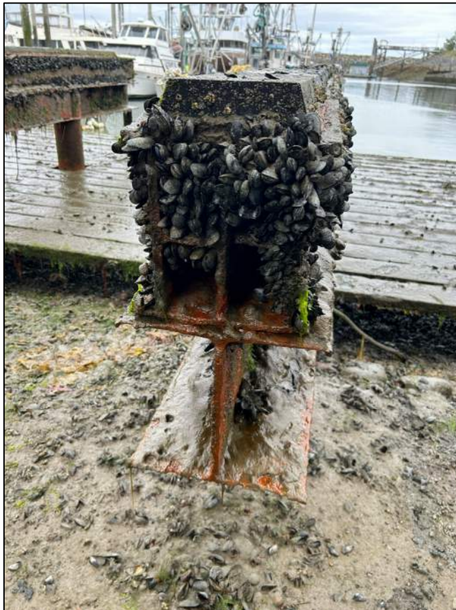
Figure 1-1. Photo of Cross-Section of Primary Structural Beams
