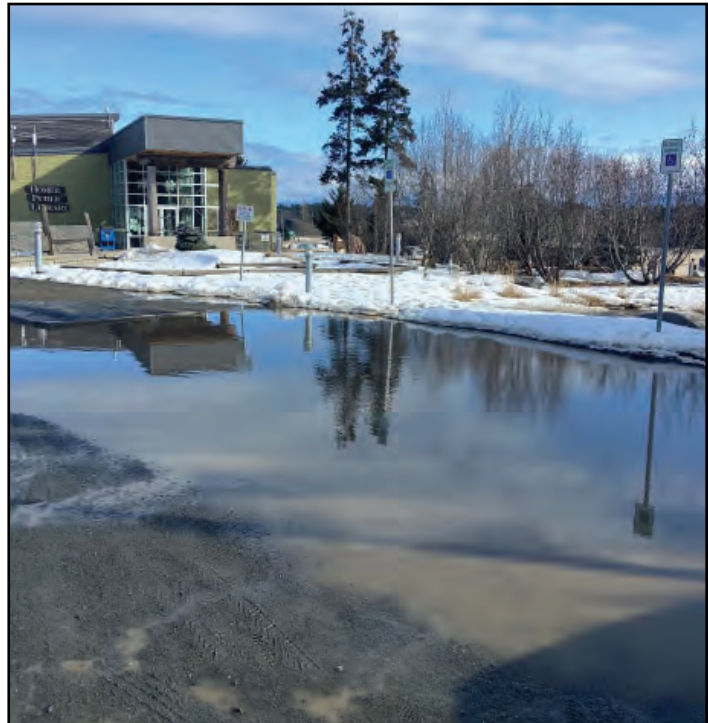
Drainage issues, especially during freeze thaw cycles in the winter and spring months create hazardous access conditions at Homer Public Library.
