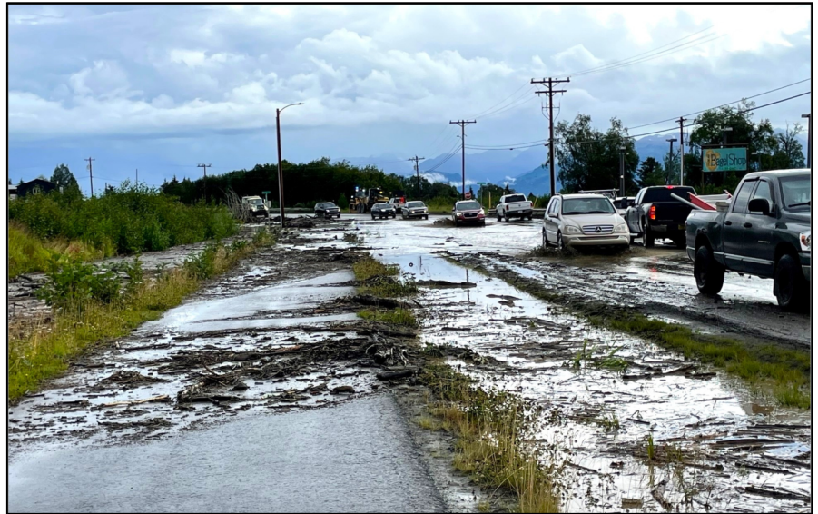
Traffic passing through the flooded section of East End Road at Kachemak Drive.
