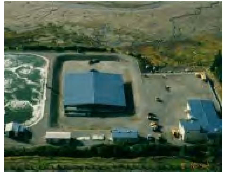
Sewer Treatment Plant, 1990
