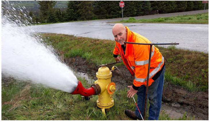
In this photo, Dave Welty is sloooowly shutting down a hydrant, as part of the City's annual hydrant-flushing program. Hydrant flushing maintains water quality by cleaning out bioslimes, manganese deposits and sediment from the water distribution mains. Opera procedures are highly choreographed and carefully
