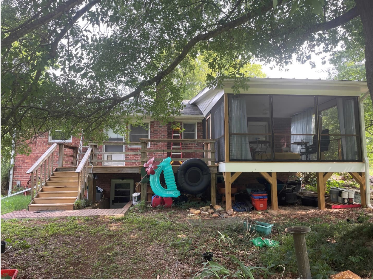
Rear (looking north)
