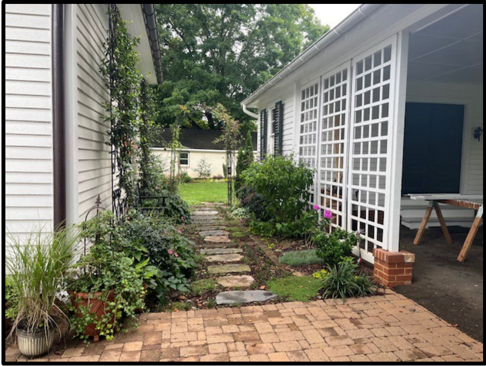
South elevation, path between carport/house
