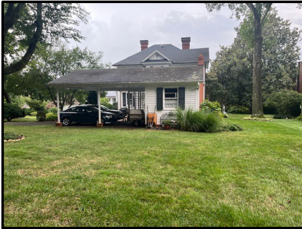
North elevation- view from backyard
