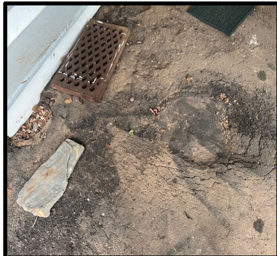
Driveway pad- asphalt with minimal or no sub-base
