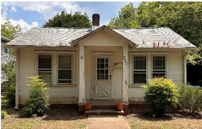
The undersized 2x4 ceiling rafters have created a dangerously sagging roof
