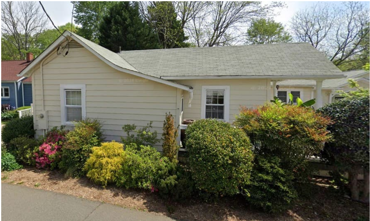
View from Lydia Lane looking East
