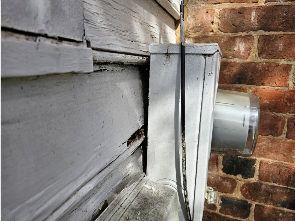
The above photo shows a section of the home that is currently using wood and Hardie siding. The below photo shows an up close section of rotted wood which can be found in nearly 50% of the siding around the home.
