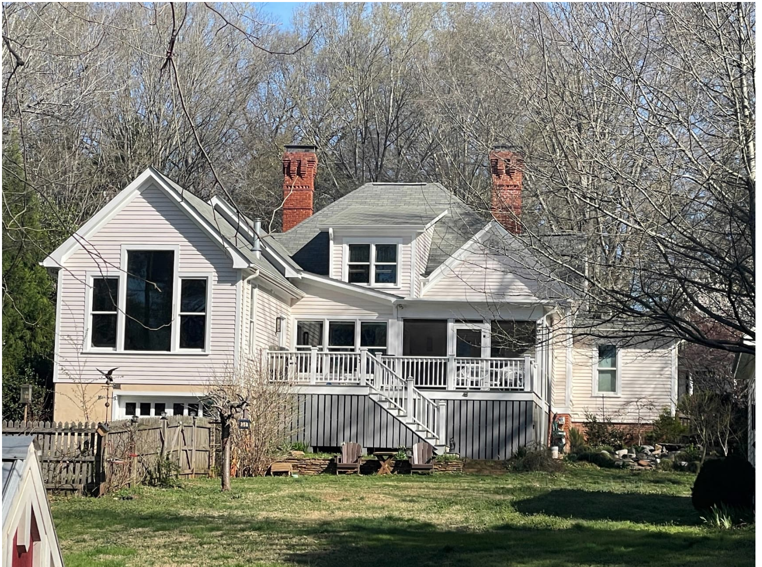
110 East Queen Street – historic house w/ rear modifications incl. similar “flat” roof screen room
