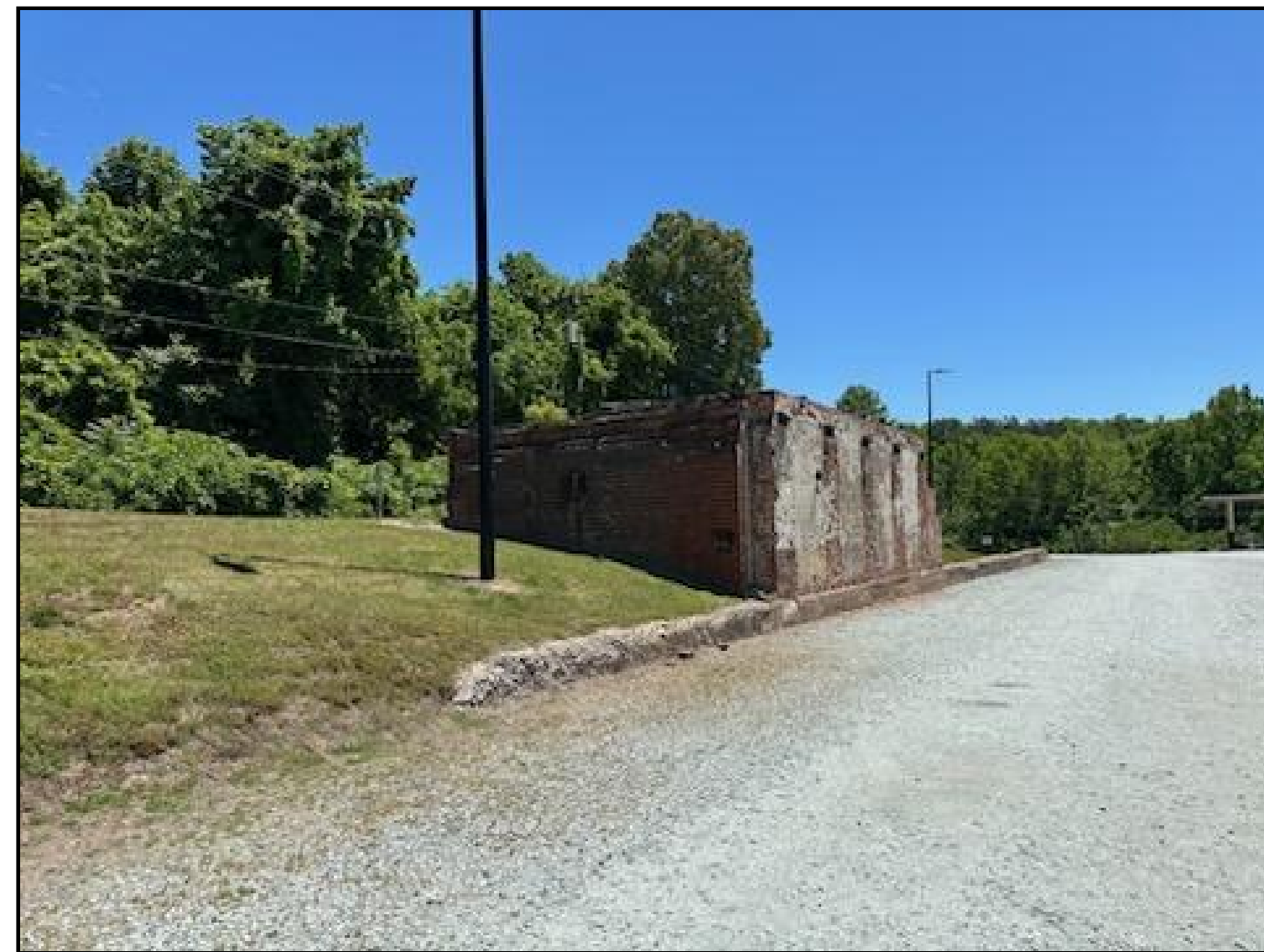
3. LOOKING SOUTHEAST TOWARDS ABANDONED OUTBUILDING
