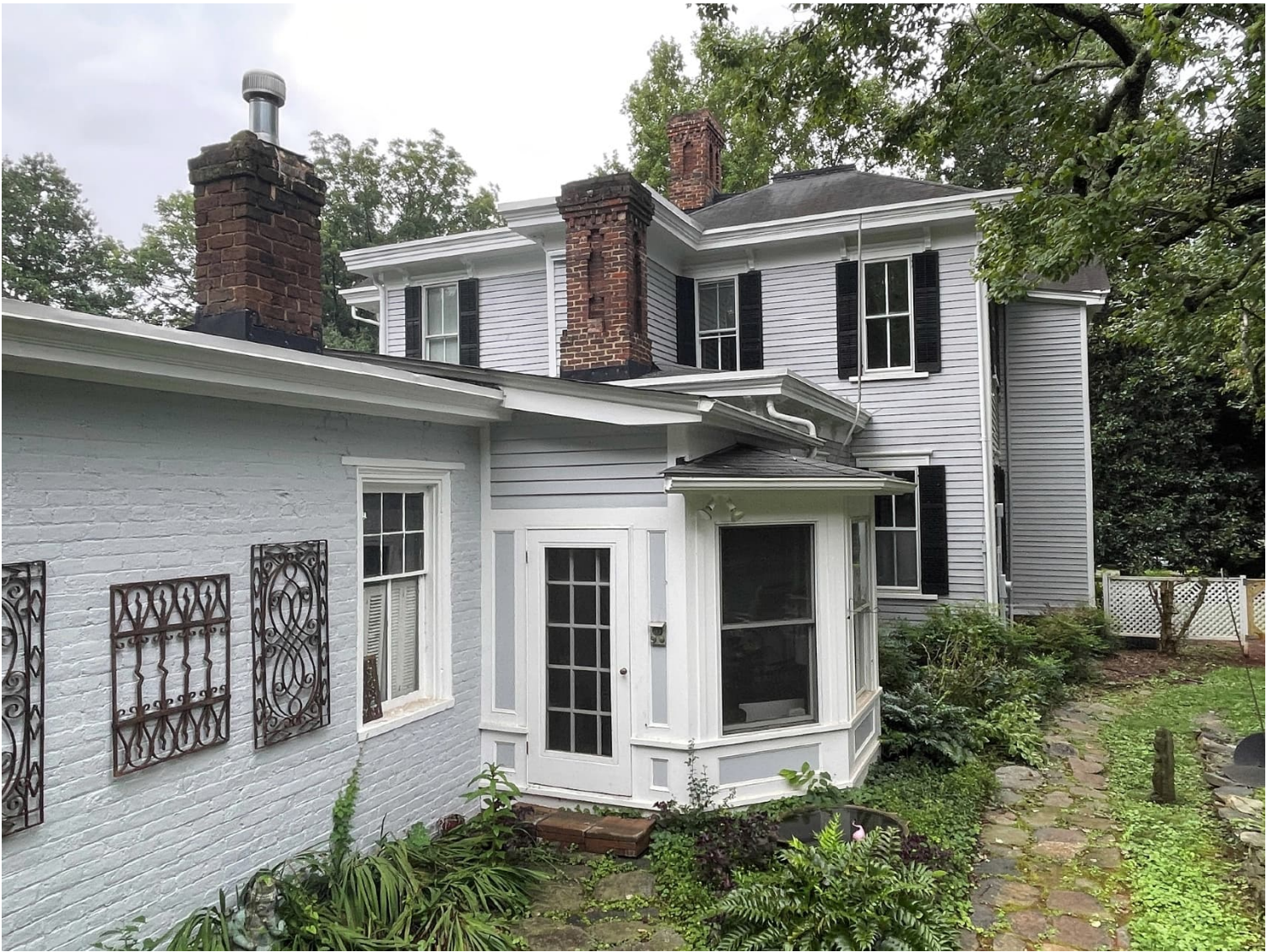
Current photo showing 1998 addition between kitchen and brick furnace building
