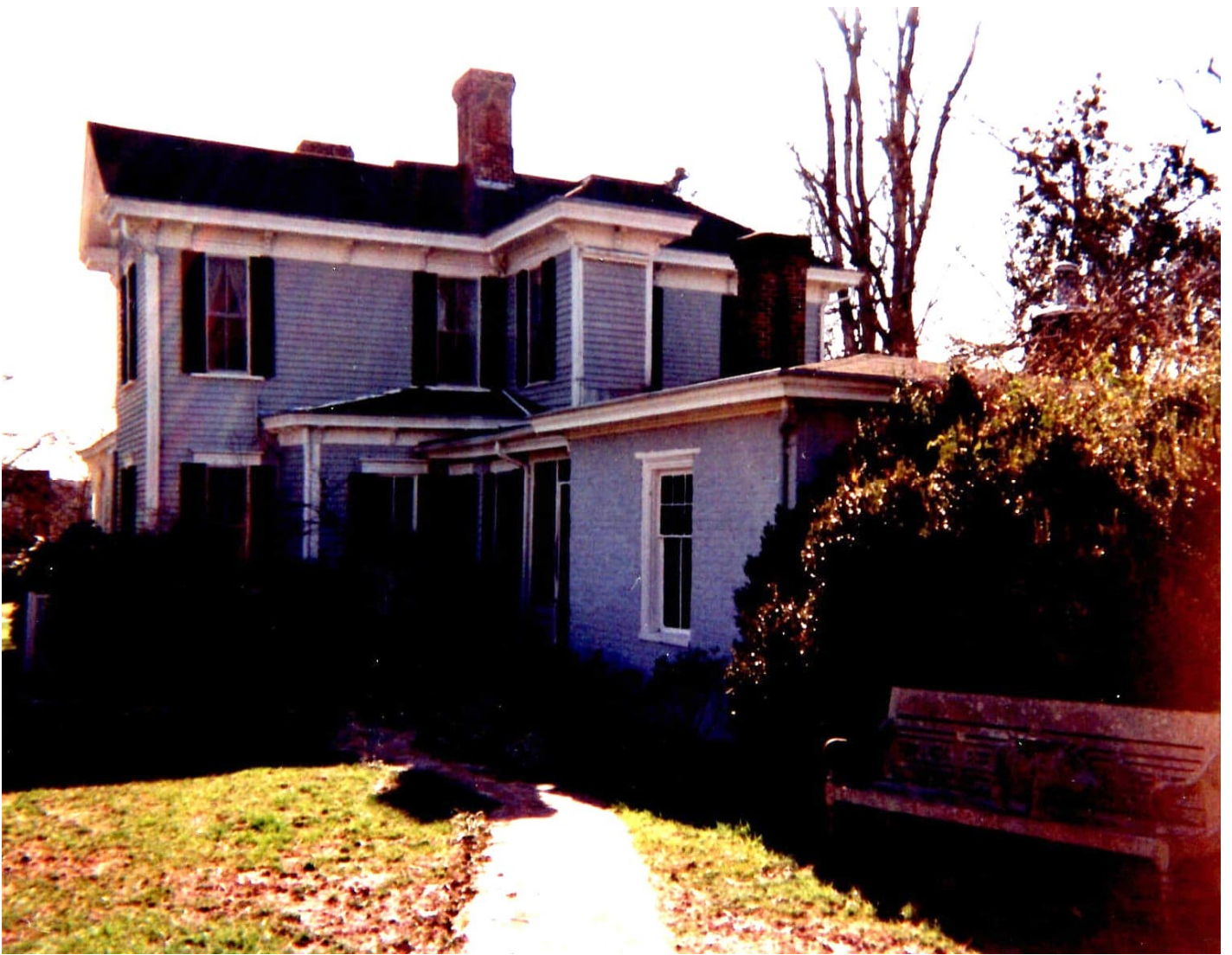
1998 photo of north elevation looking southwest prior to renovation
