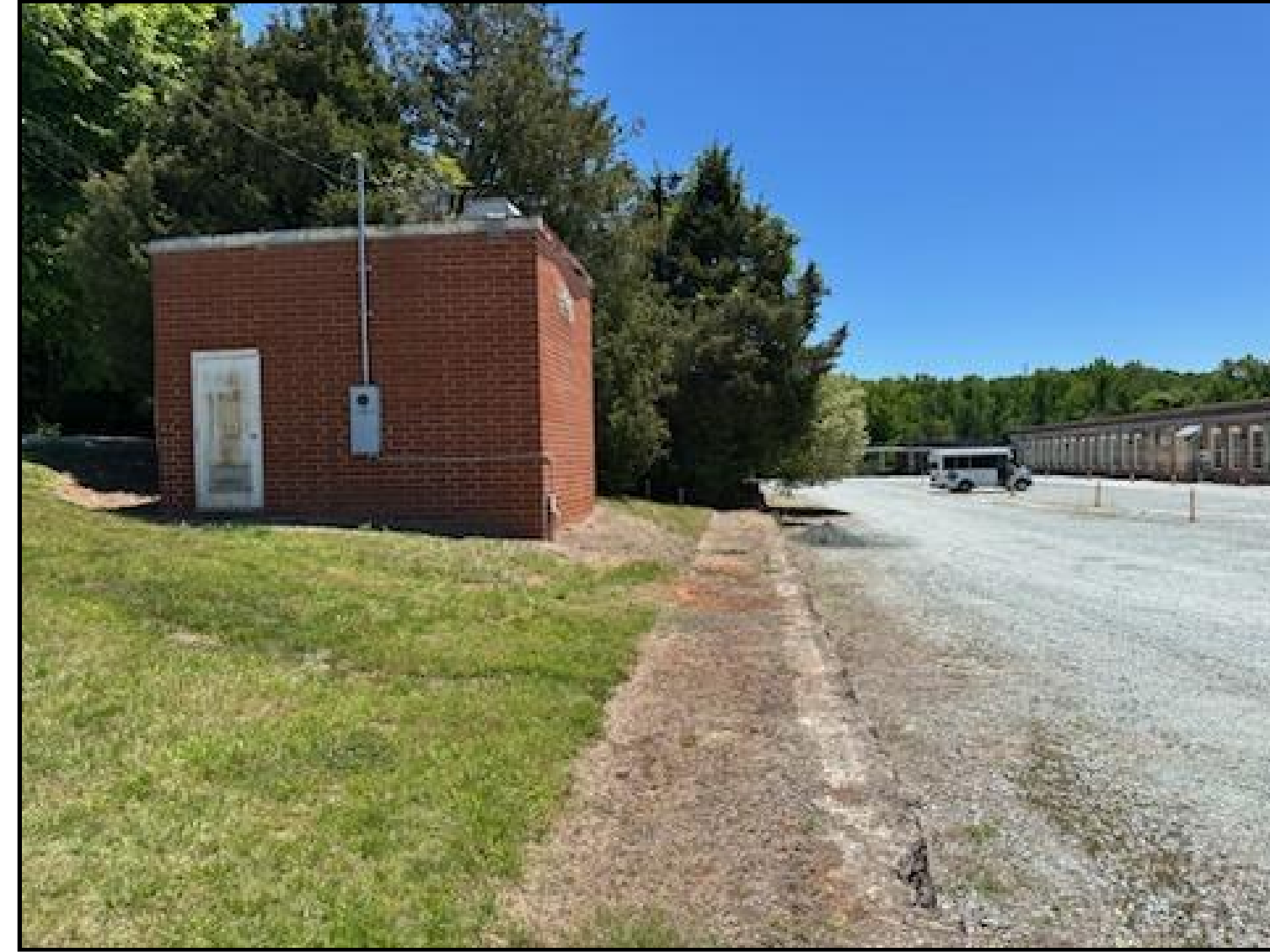
1. LOOKING SOUTH TOWARDS GRAVEL LOT
