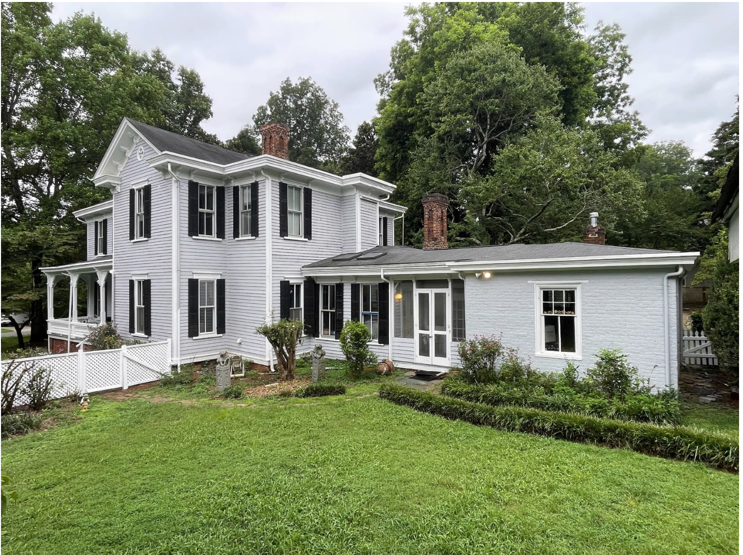
Current photo of northeast elevation showing 1998 2 nd story bathroom addition & 1 st story roof modification
