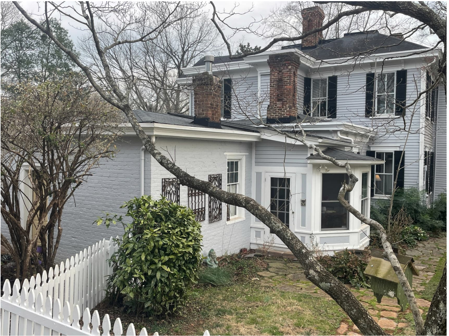
Current photo of rear elevation looking south
