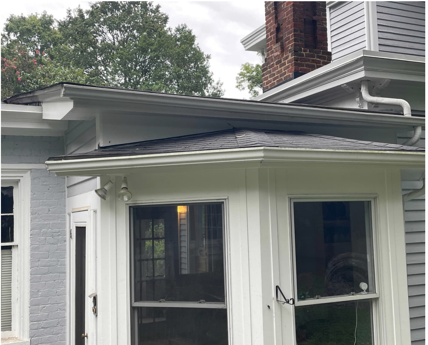
Current photo showing intersecting rooflines
