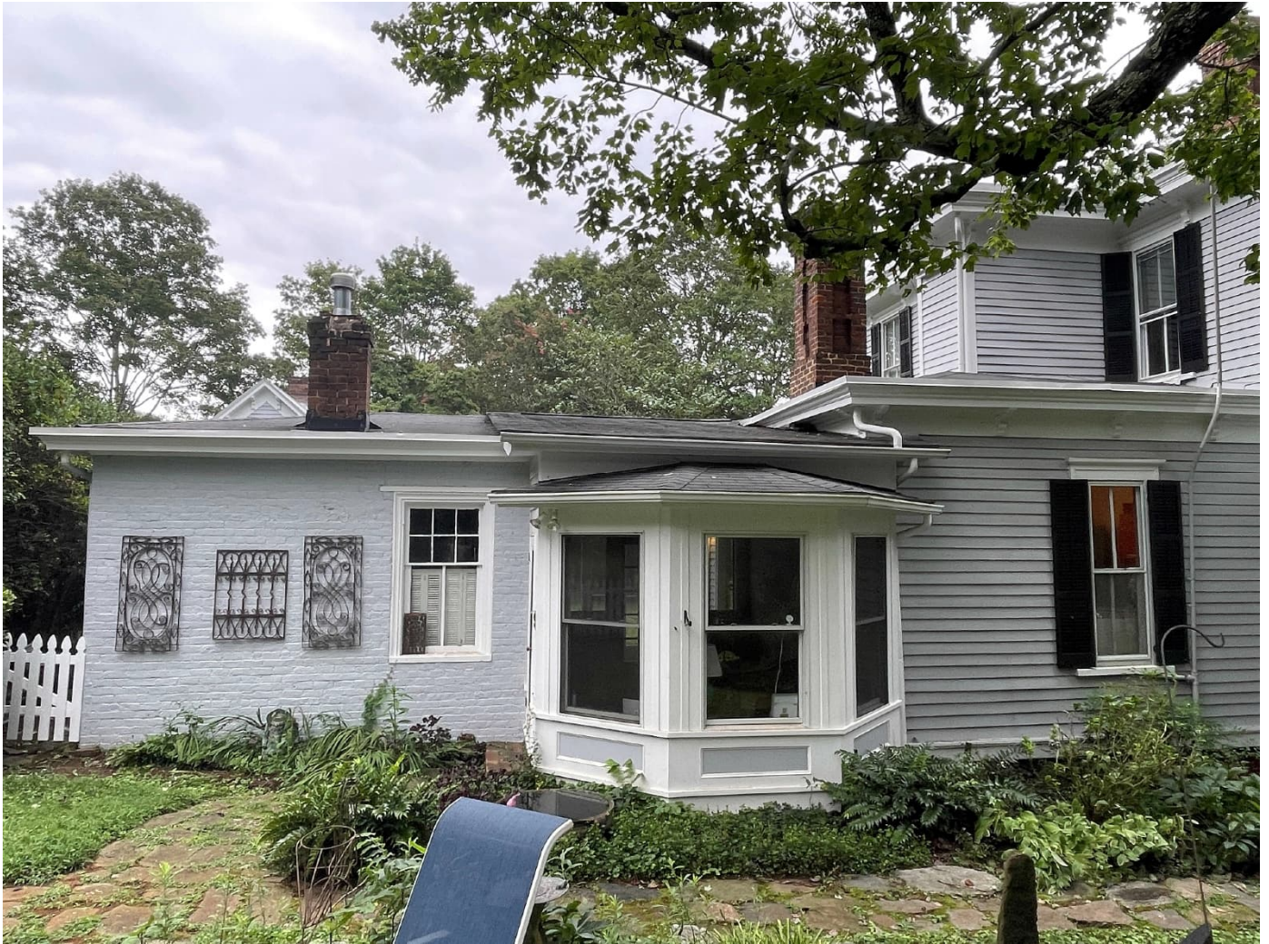
Current photo of west elevation showing 1998 addition between kitchen and brick furnace building
