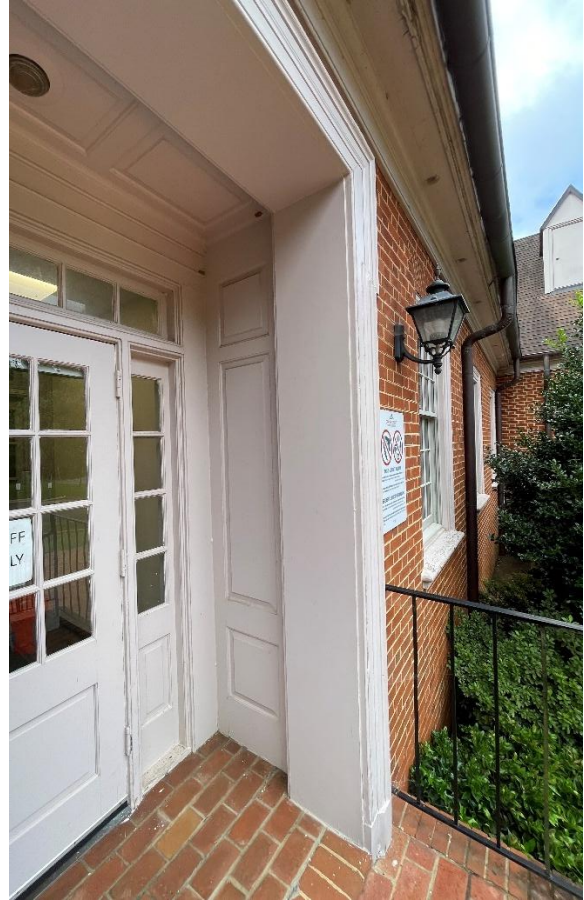
Existing rear entrance to be reused or emulated Light fixture detail. Round copper gutter and downspouts
