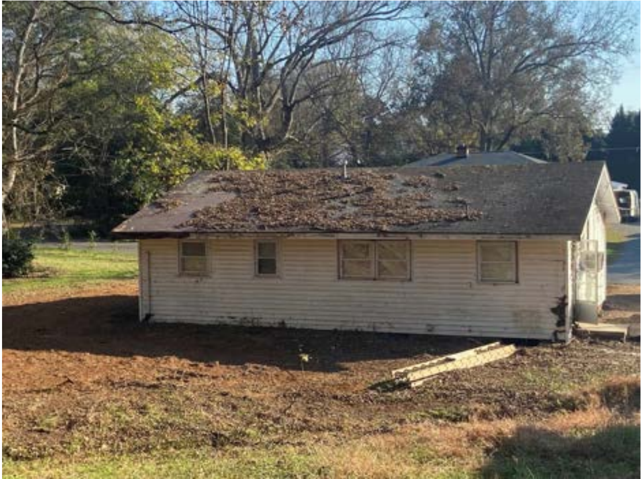
Rear/North- proposed rear addition with asphalt shingles and brick foundation to match, wood windows, fiberglass patio door, Hardie siding, Miratec trim and wood decks
