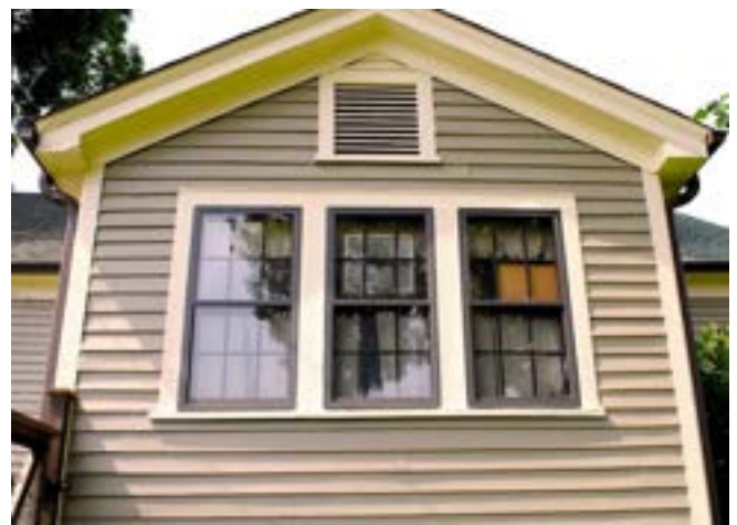
The frames and panes of the storm windows at 216 S. Hillsborough Ave. match the divisions of the window underneath.
