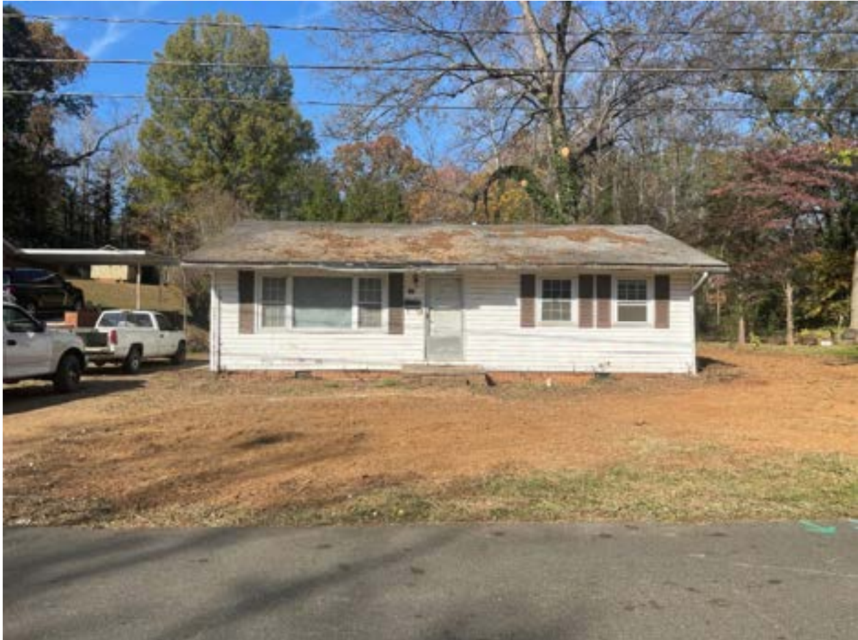
Front/South (facing W Union St) – proposed replace vinyl windows with wood windows, existing vinyl siding/trim to remain and new wood columned stoop with asphalt shingles, Hardie siding/Miratec trim
