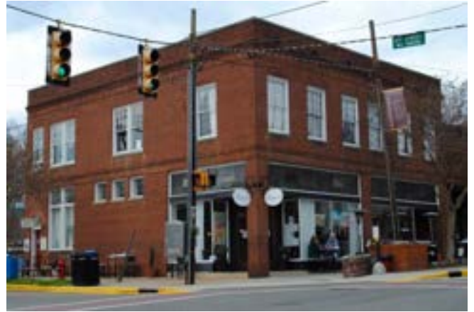
Flat roofs and high parapets of commercial buildings provide an opportunity for the discreet placement of mechanical units.
