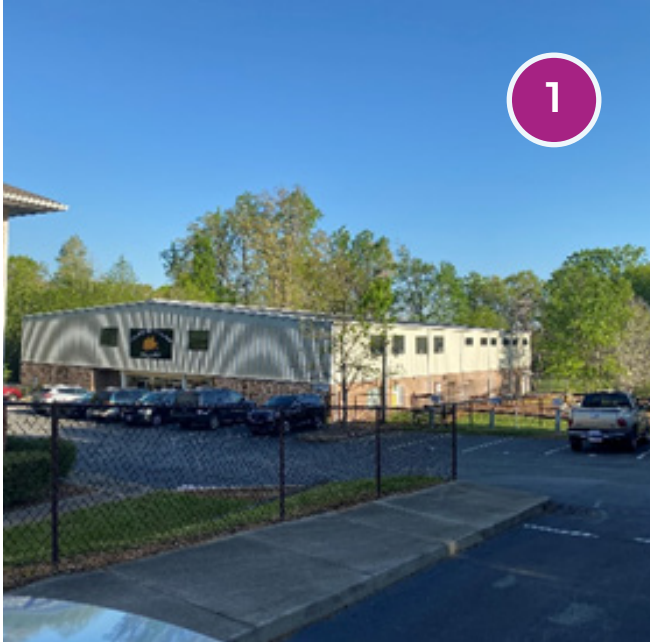
School campus and parking lot
