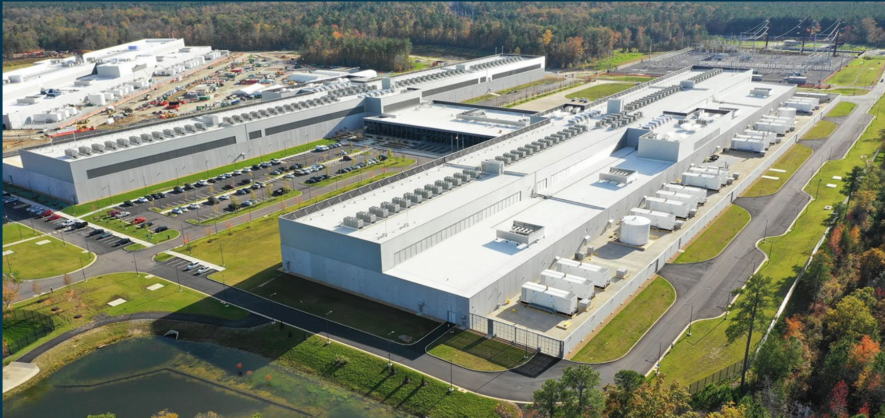
Source: DPR.COM Meta's Henrico County Data Center
