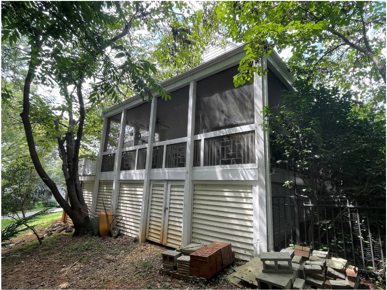
View of right side (east elevation)
