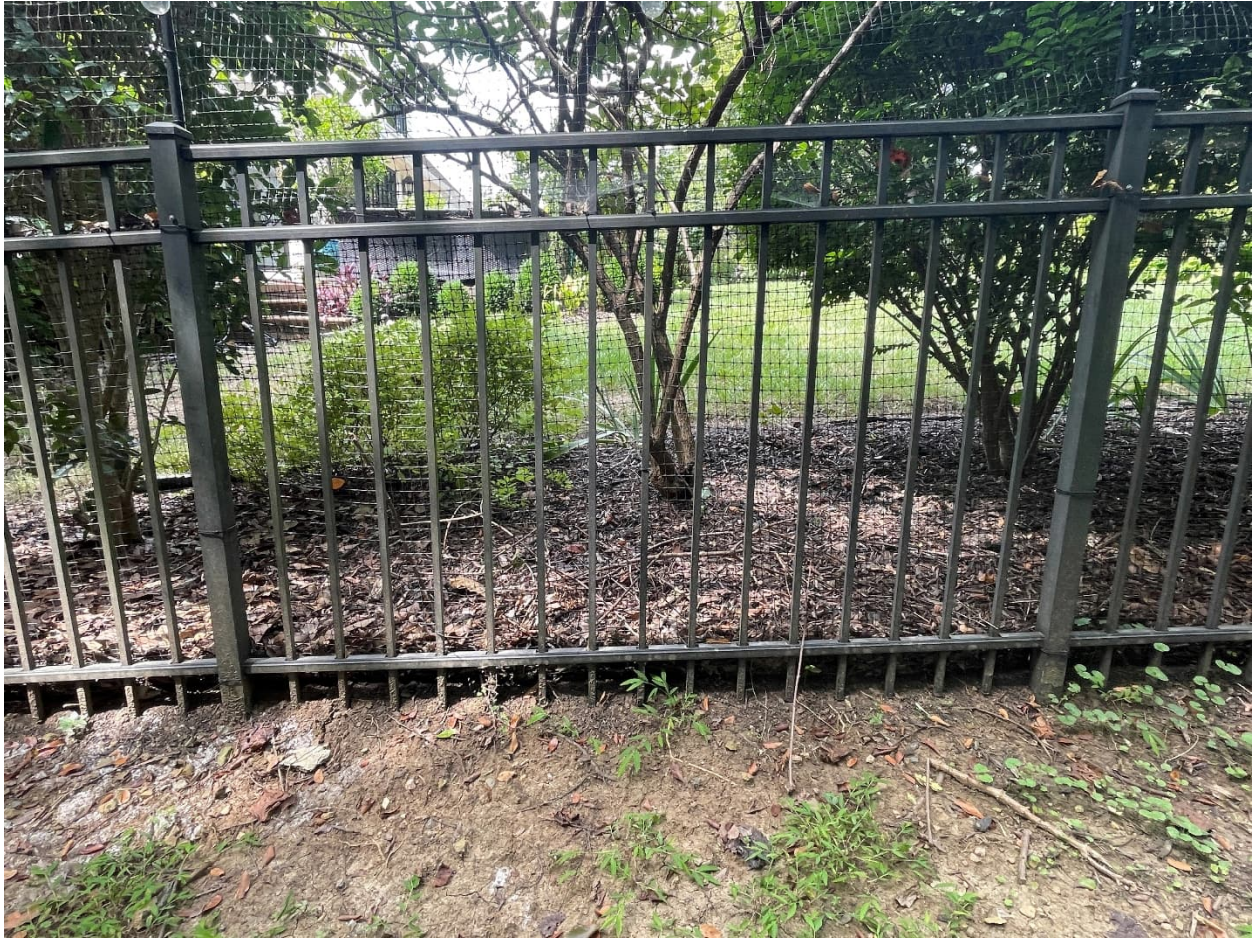
View of existing metal fence to be adjusted to accommodate proposed pool
