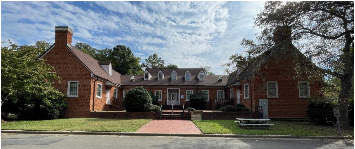
Overall west elevation (building rear)
