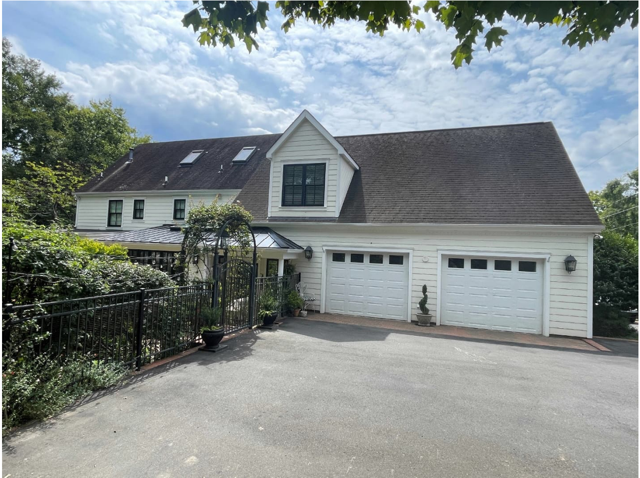
View of rear (north elevation)
