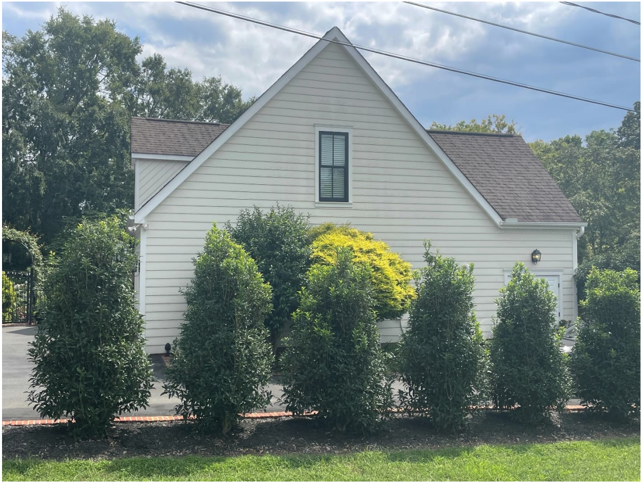
View of left side (west elevation)
