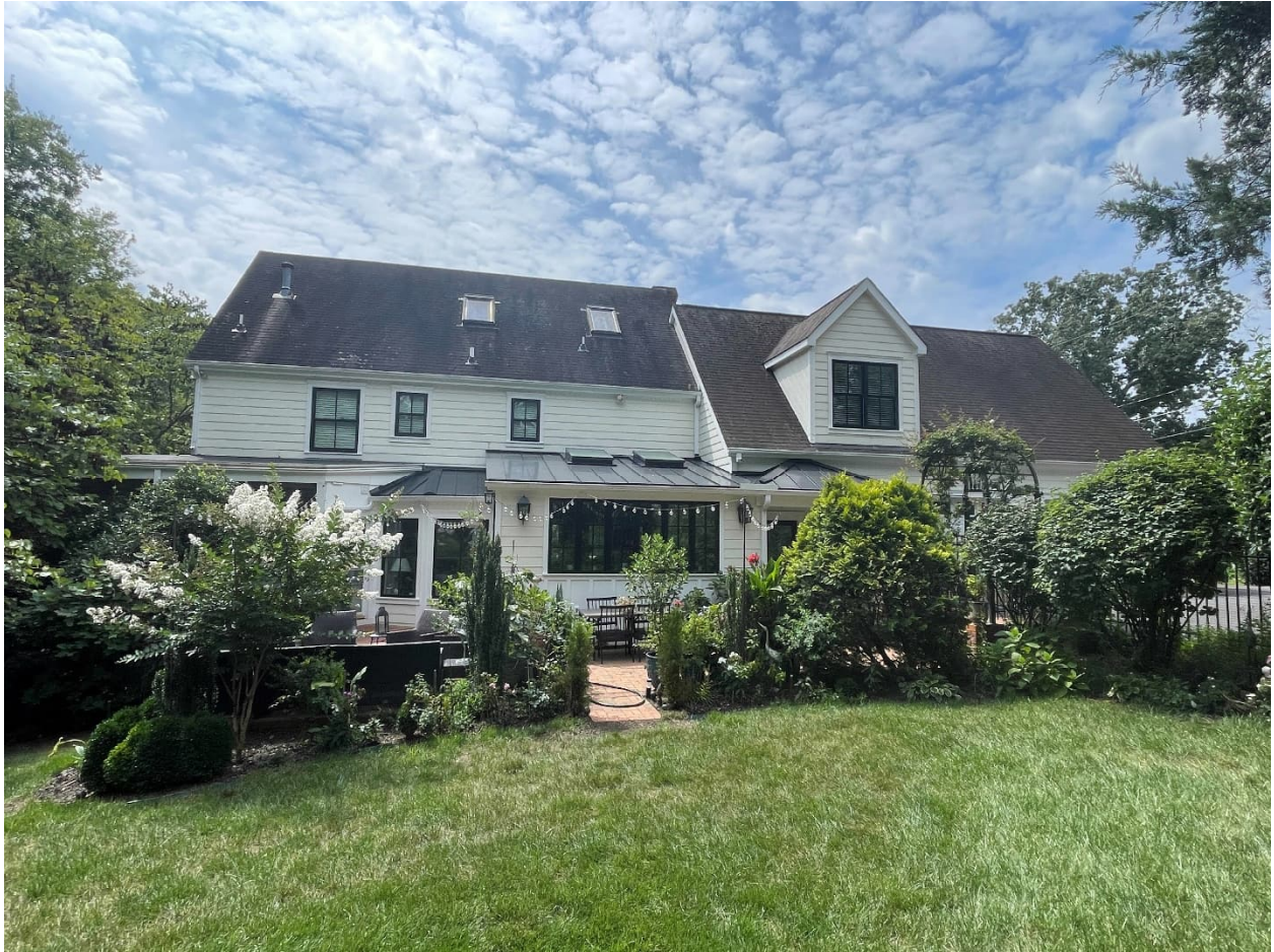
Additional view of rear (north elevation)
