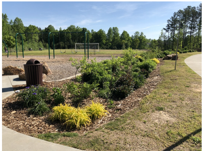
Stormwater retrofit linear pollinator garden
