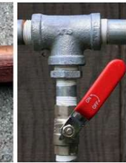
Galvanized Steel and Valve
