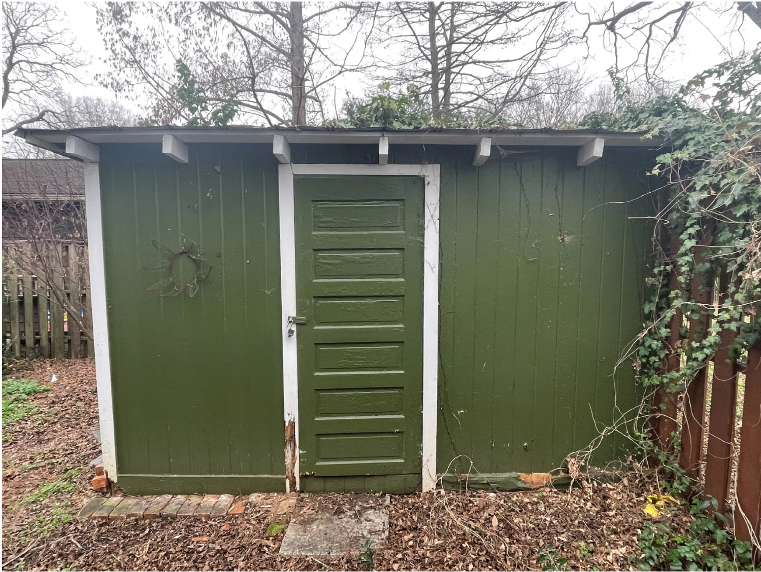
Shed Right Side looking south
