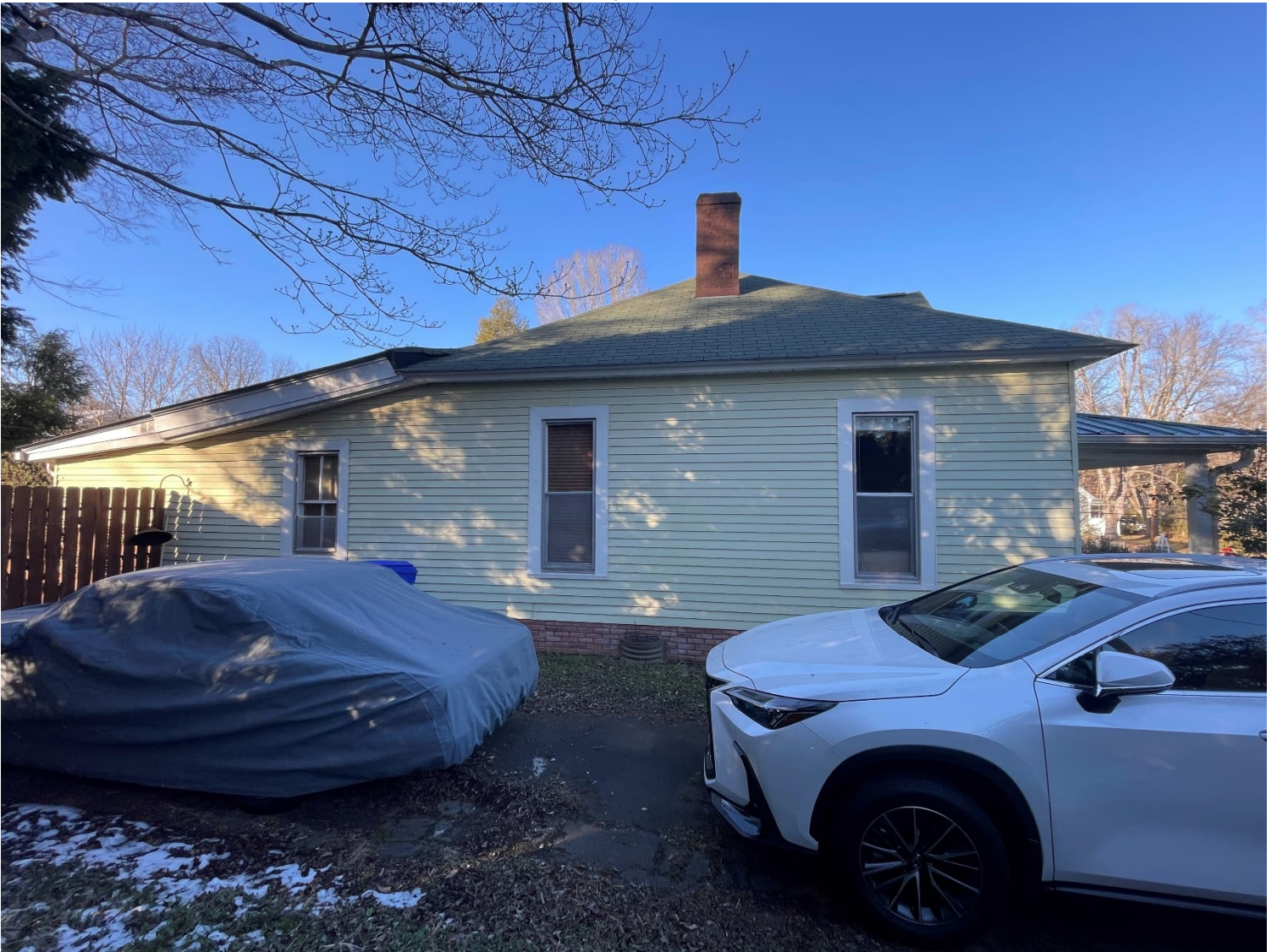
Left side looking north
