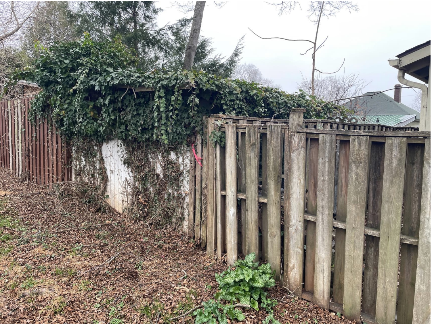
Left side obscured and inaccessible for photos
