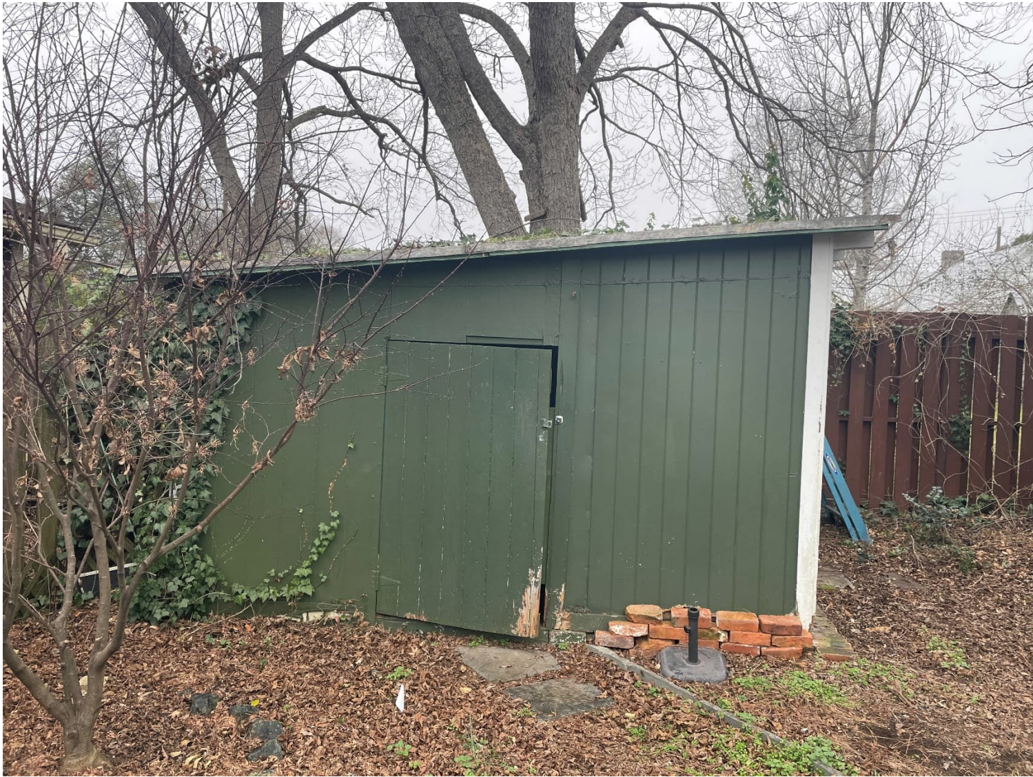
Shed Front looking west
