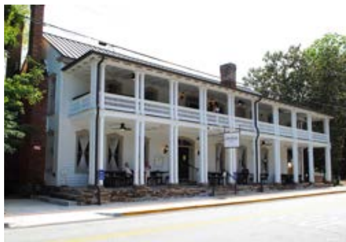
The Colonial Inn at 153 W. King St. was rehabilitated in 2020 using historic tax credits after standing vacant for almost 20 years.
