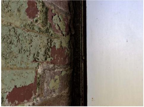
Asbestos containing window caulk between window sash and brick.
