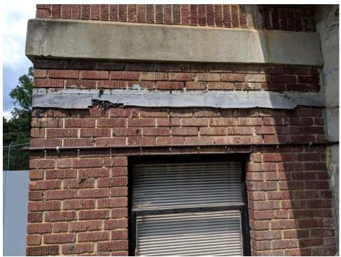
Asbestos containing flashing on C Side.
