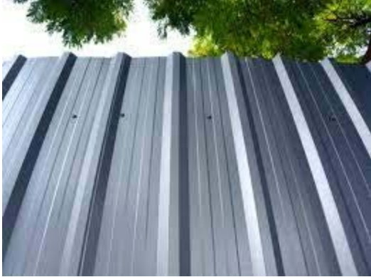
Corrogated metal roof example.
