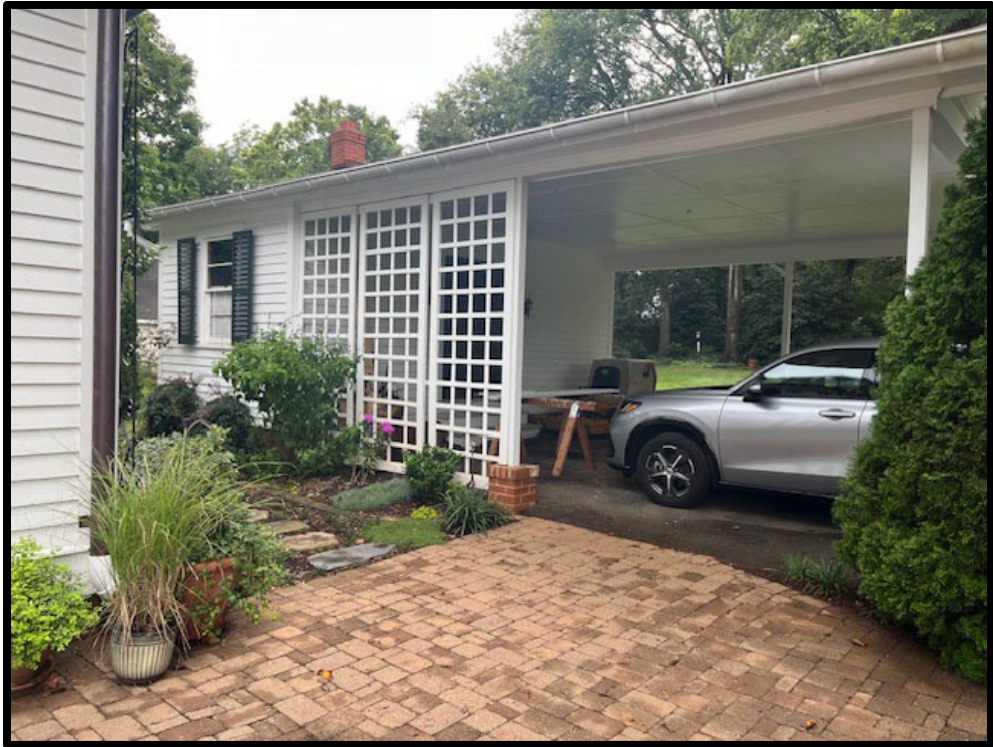
South elevation, view from patio
