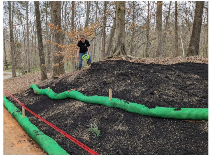
Compost Blanket Installation
