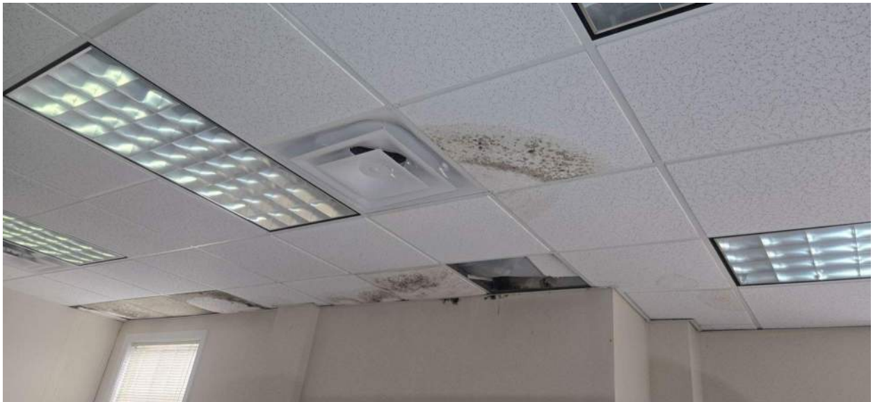
Photo 4: Condition of Room 241
