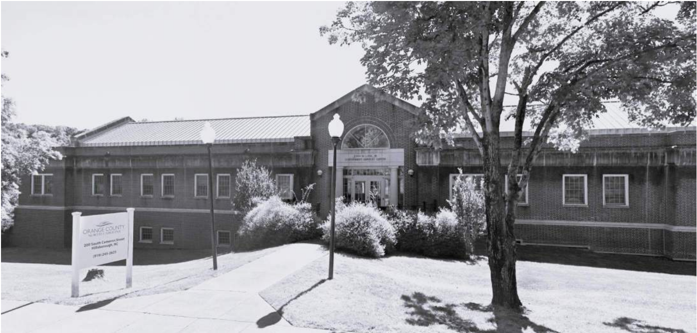
Existing Building Conditions
