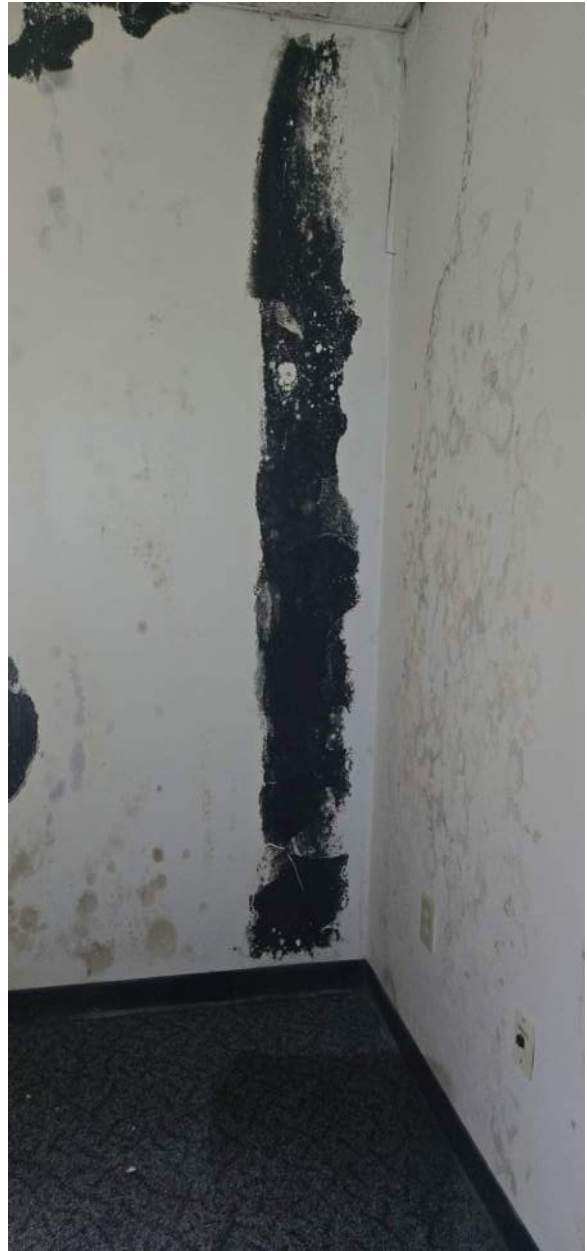
Photo 2: Condition of basement.
