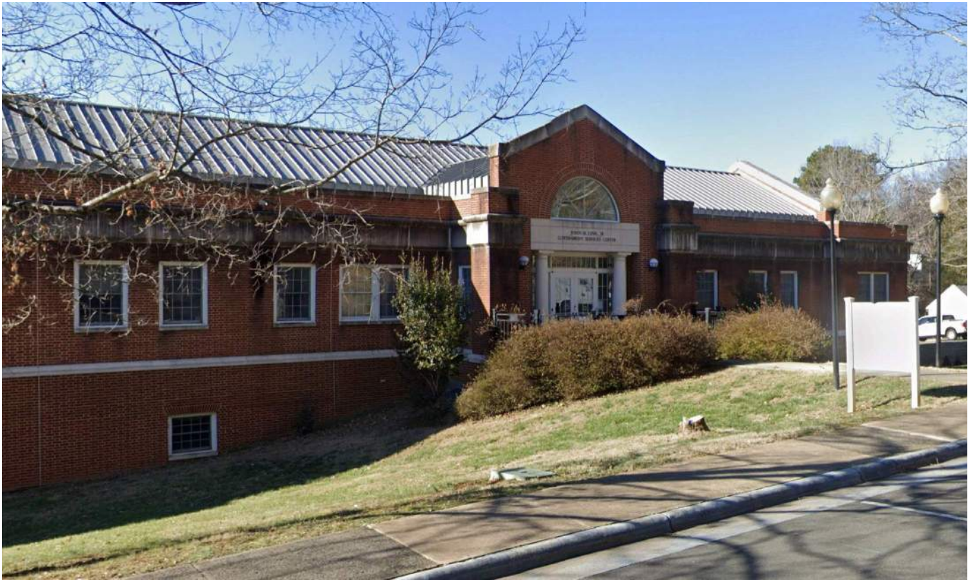
Building entry- S. Cameron St.
