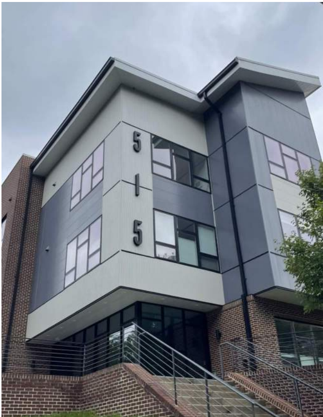
Apartments at 515 N Churton St
