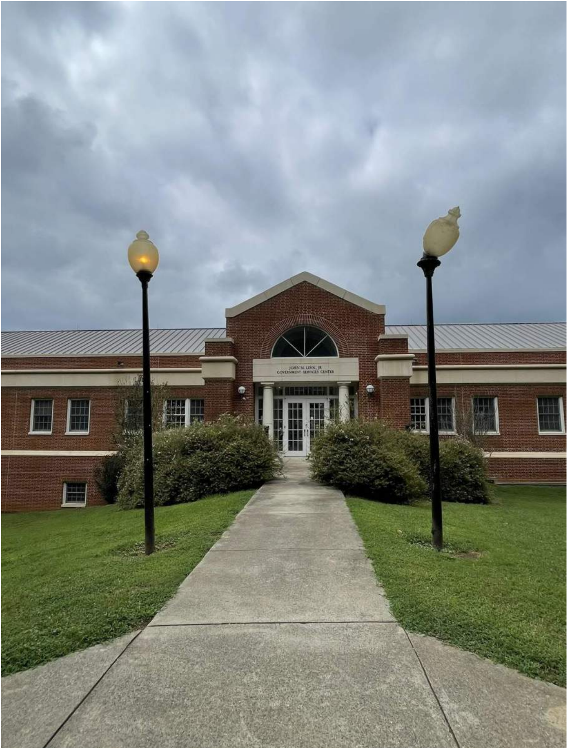
Building entry- S. Cameron St.
