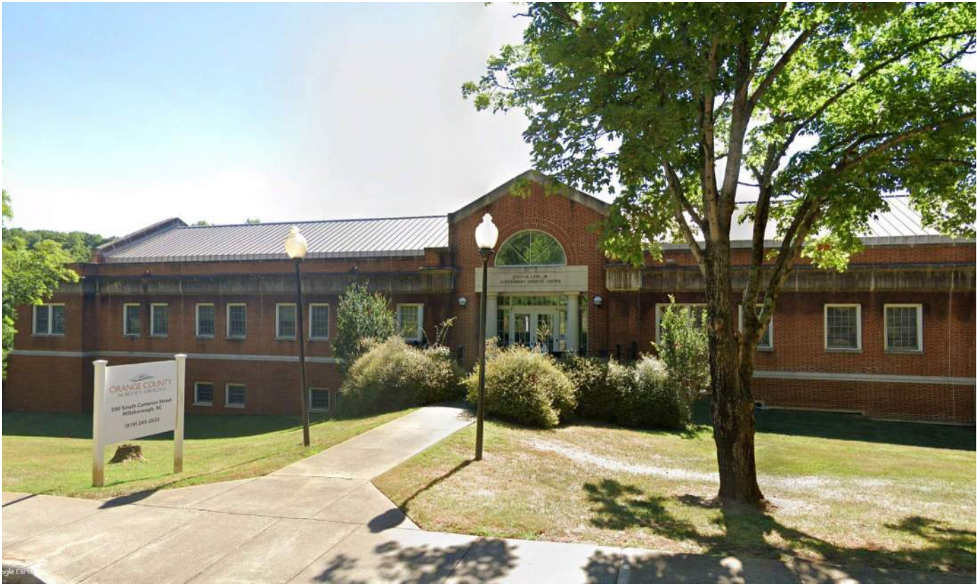
Building entry- S. Cameron St.
