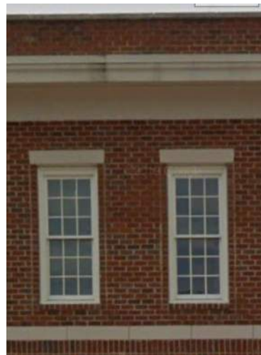
Orange County West Campus Offices
