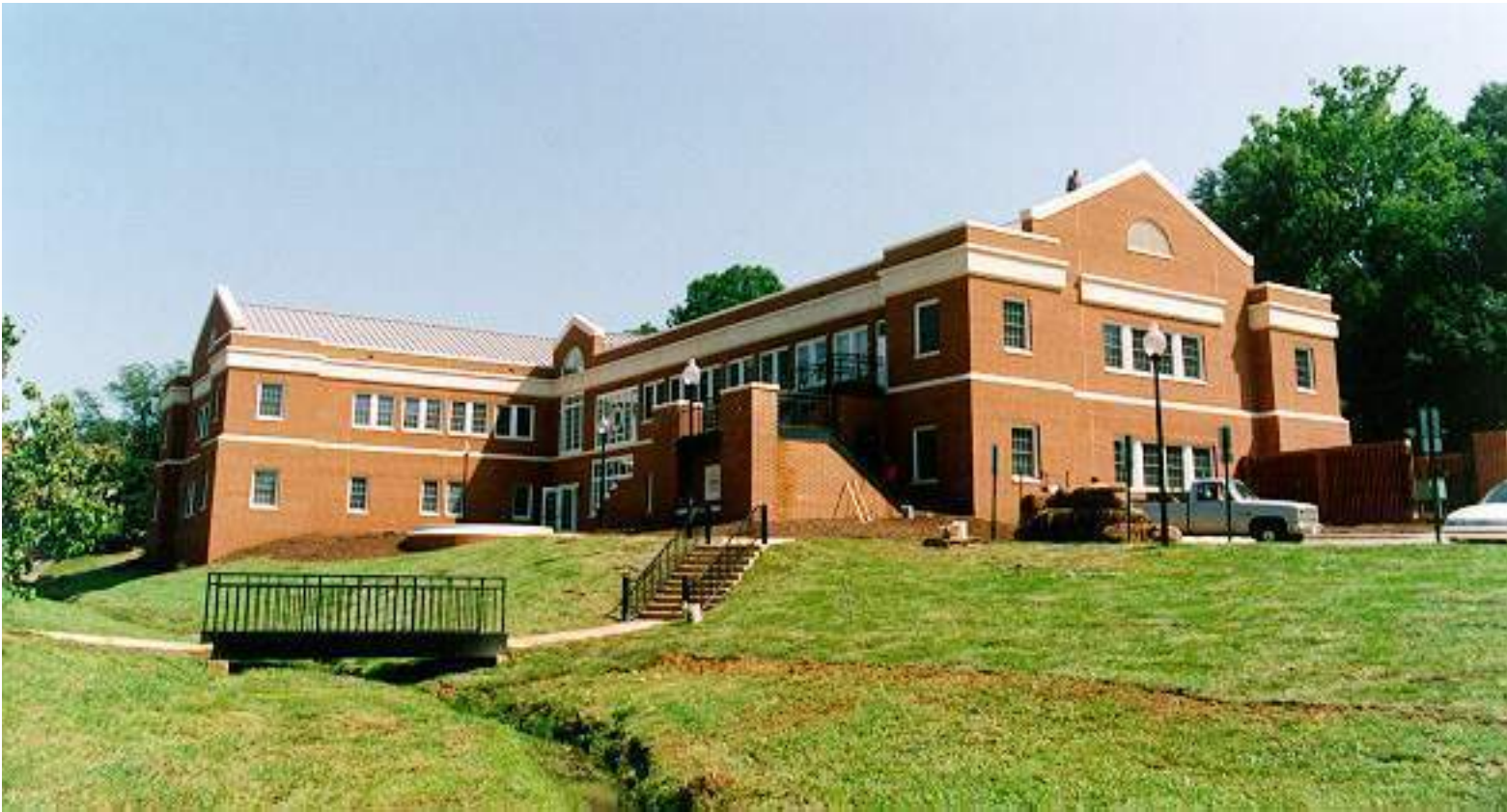
Exterior view of Link Building- Prior planting near stream
