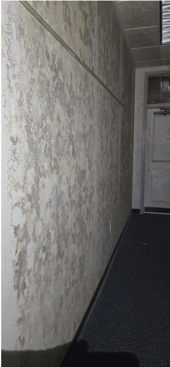
Photo 1: Condition of basement @ sample 1.
