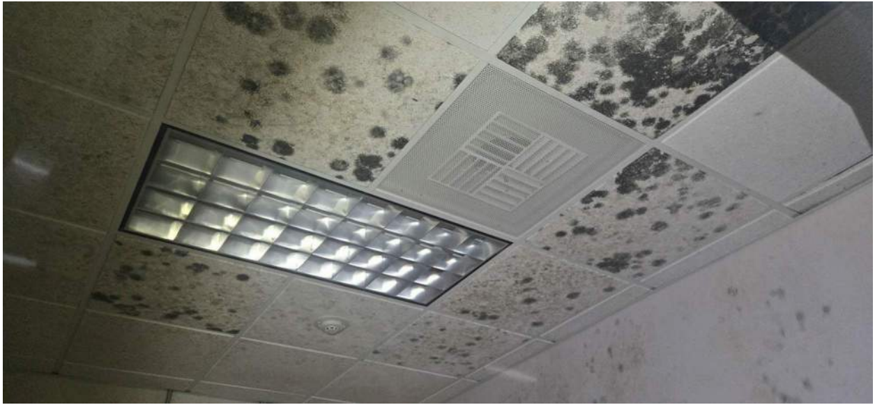
Photo 3: Condition of basement.
