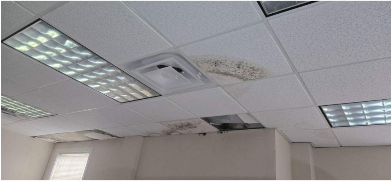
Photo 5: Condition of Room 241
