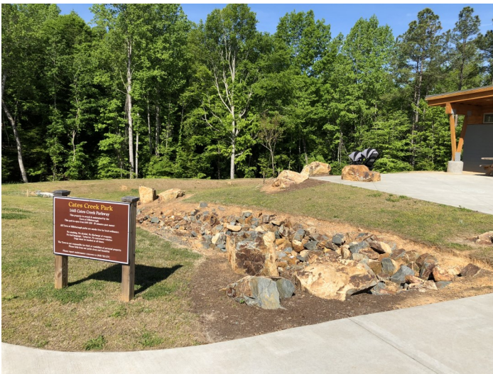
Stormwater Control Measure
