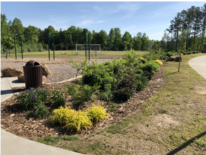
Stormwater retrofit linear pollinator garden
