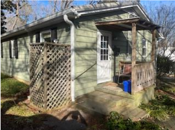
Existing Exterior Hot Water Heater Enclosure w/Lattice Screen
