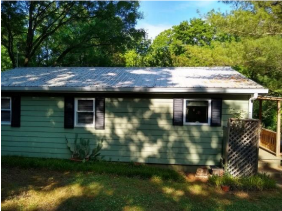
Existing Roof Material – “Master Rib” metal roofing
