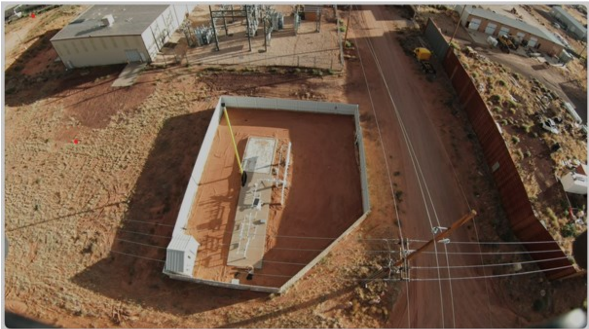
Aerial view of the Hildale Natural Gas Gate Station
