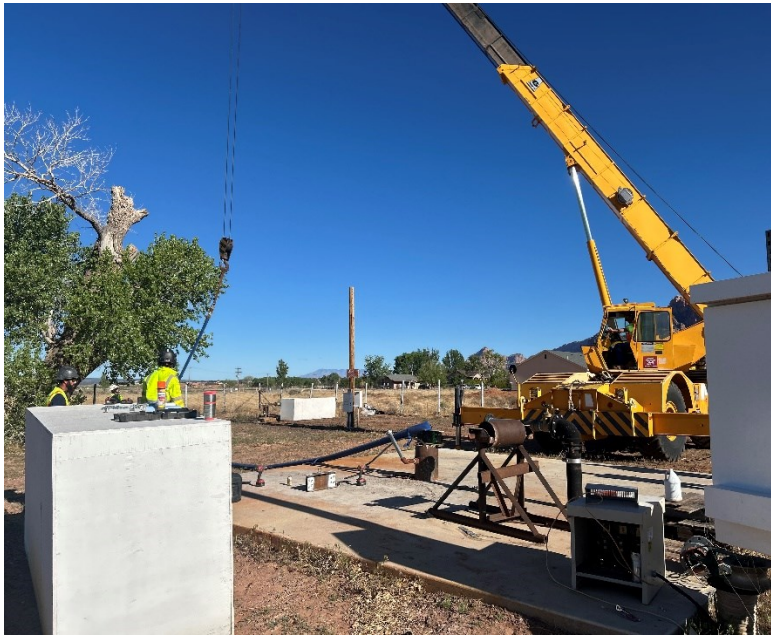
(Crew Pulling the Pump and Motor)
