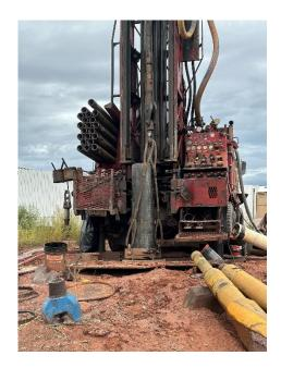
Cluff drilling continues to drill replacement Well 17 and have installed casing to the depth of 560 feet. To date the well has been drilled to over 600 feet in depth.
