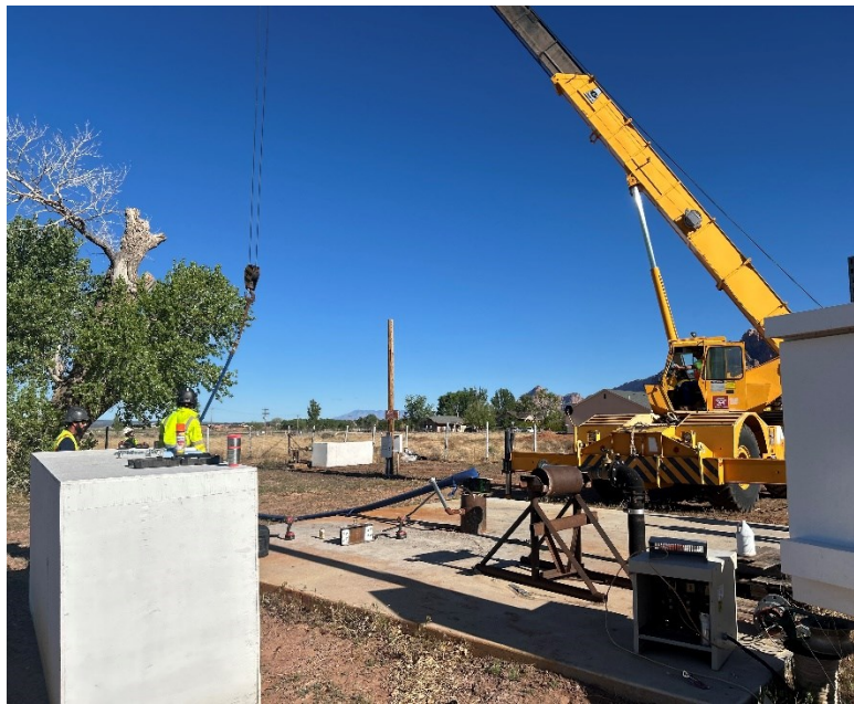
(Crew Pulling the Pump and Motor)
