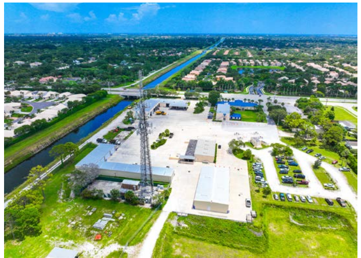
[LWDD Headquarters, Delray Beach, FL]
