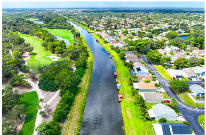
[Lake Worth Drainage District, Lake Worth, FL]
