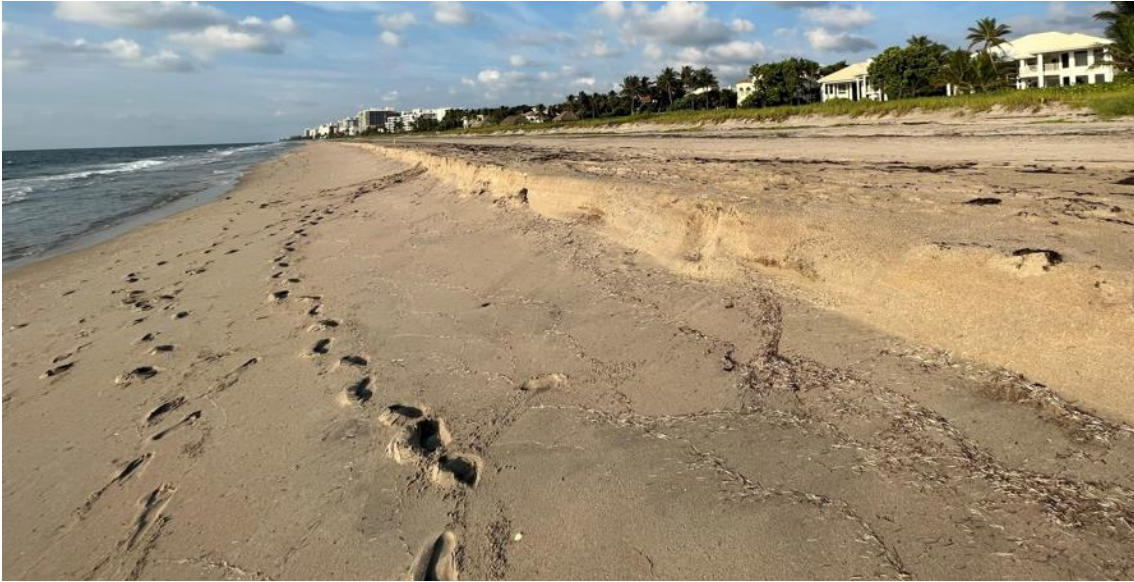
Photo 1. View looking south at the Highland Beach-Delray Beach municipal boundary. The berm has an approximate 20-inch scarp which diminishes to the south.
