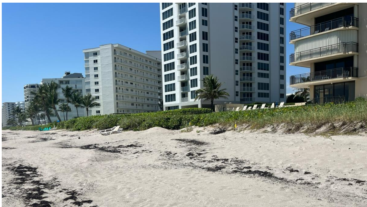
Photo 3. (From right to left) The scarped dune toe in front of Ocean Pines Condo. The scarped dune toe is hidden behind the seagrasses in front of Ocean Dunes Condo.
