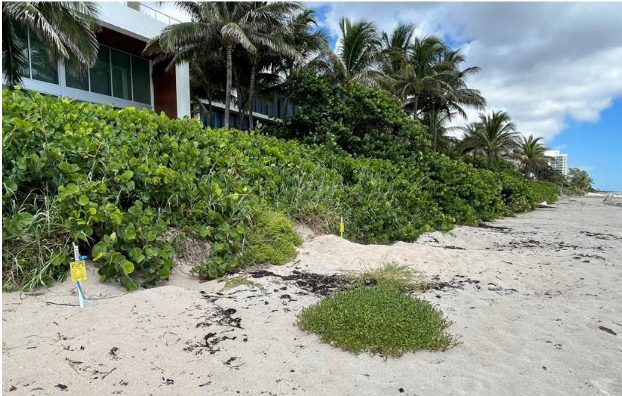
Photo 8. Dune face scarping is resulting in undermining of the dune vegetation 1 in front of 3715 South Ocean Boulevard.
