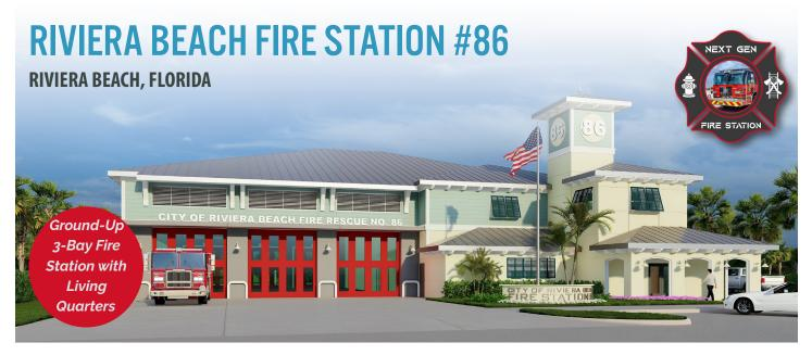
New construction of a two-story, 13,000 SF fire station using a HOT Zone facility layout. The project consists of three apparatus bays, sleeping and private restroom facilities for male and female firefighters, and circadian lighting.
